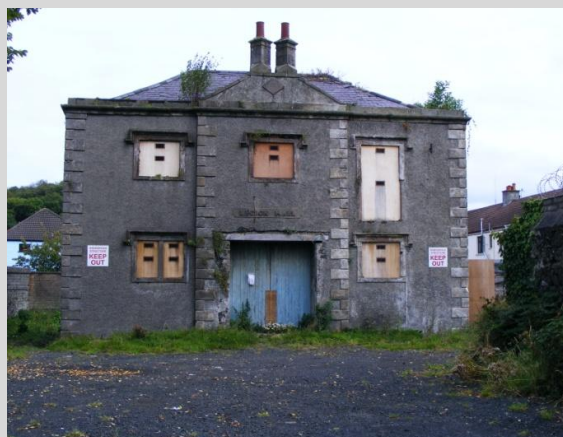
After: Openings secured, ventilation holes provided and vegetation removed
