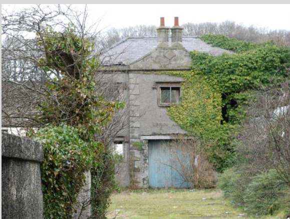
Before: Building unsecure with extensive vegetation growth
