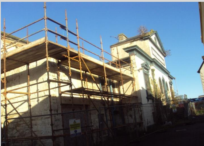
Left: Before- Sections of missing slates forming large holes to roof with openings unsecured. Above: Urgent repair works in progress to cover roof with corrugated tin and secure openings
