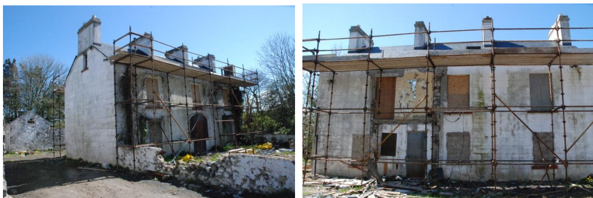
Above: Urgent Works nearing completion, Corrstown House, Portrush © DfC
