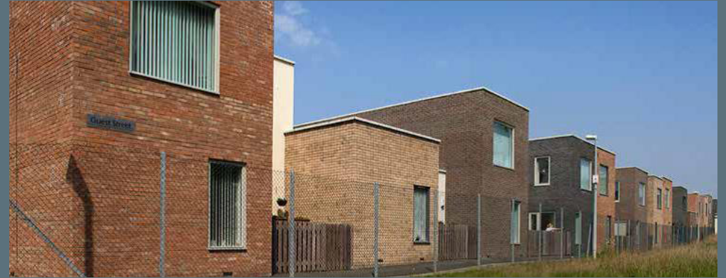
Rear return of a former terraced block following remodelling works
