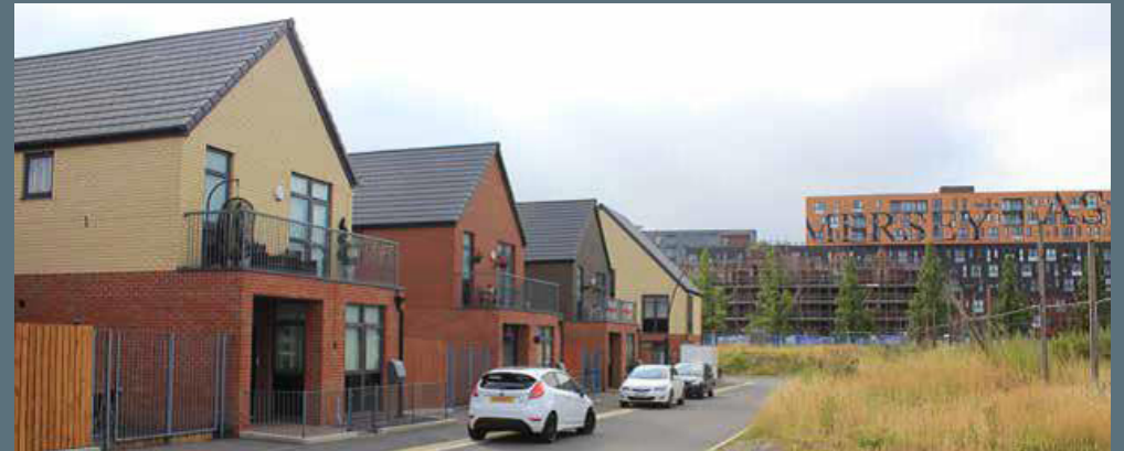
Another example of reconfiguring an existing terrace street. Properties were rotated 90 degrees, accommodating the required parking and garden space alongside the house rather than in front or behind.
