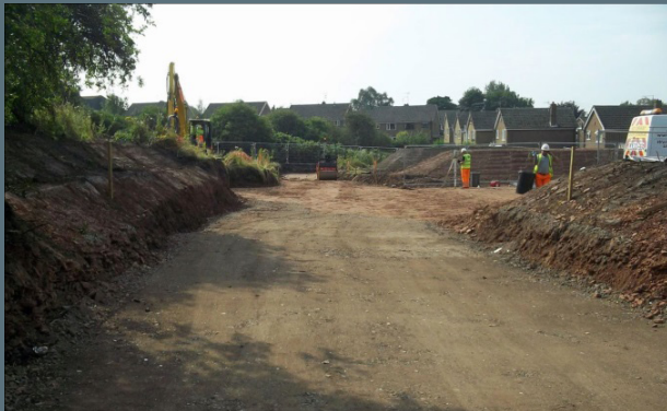
Enabling building works Sourced from Stoke-on-Trent City Council
