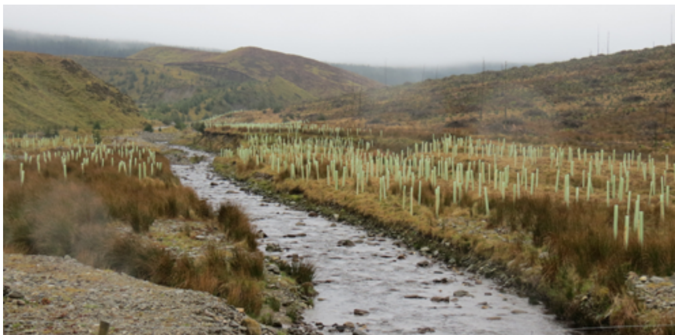
NI Water, The Woodland Trust and The Loughs Agency collaborated on a SCAMP project to stabilize the banks of Glenedra River by undertaking the planting of 5,742 native broadleaf trees in a riparian zone along the river.
