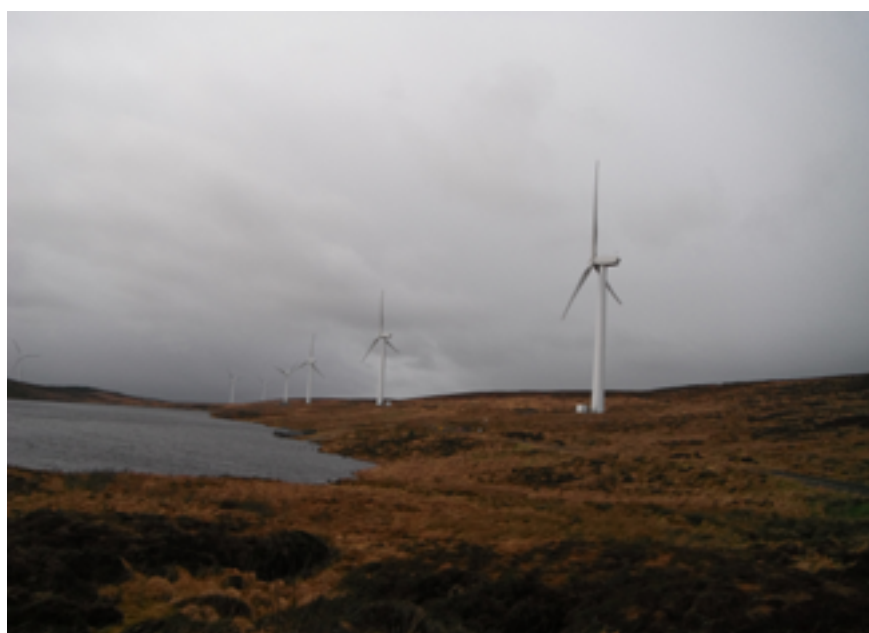
Windfarm construction adjacent to Lough Lee, in the catchment of Lough Bradan WTW
