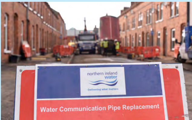
Lead communication pipes being replaced.
