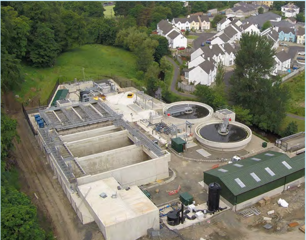
Construction of Ballycastle wastewater treatment works, Co Antrim.
