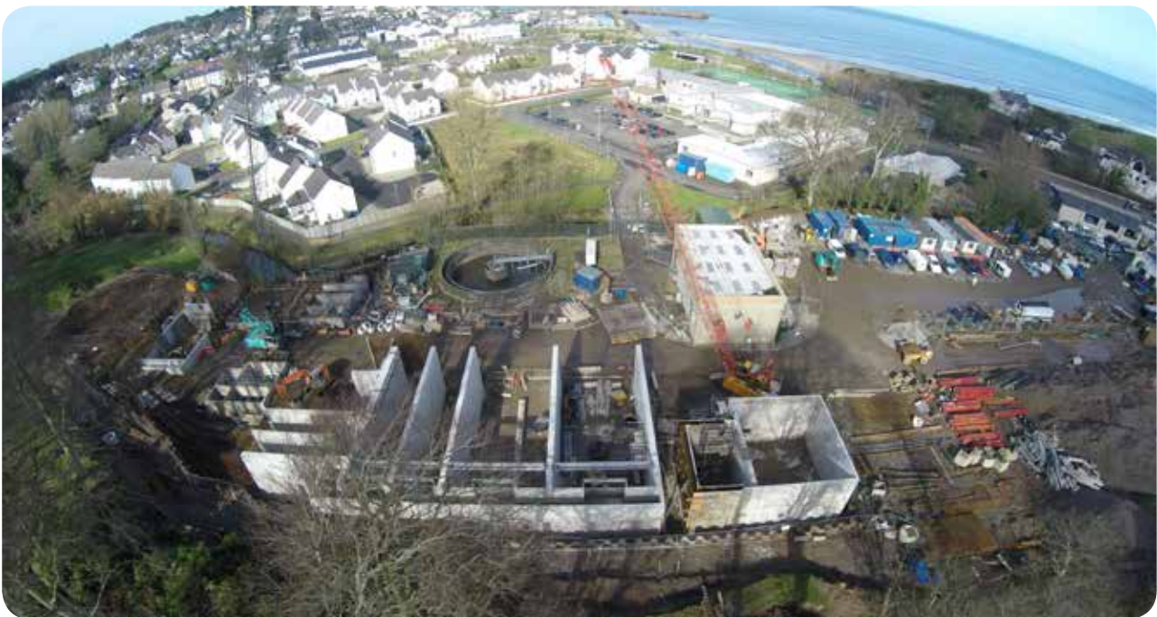
Construction of Ballycastle wastewater treatment works, Co. Antrim.
