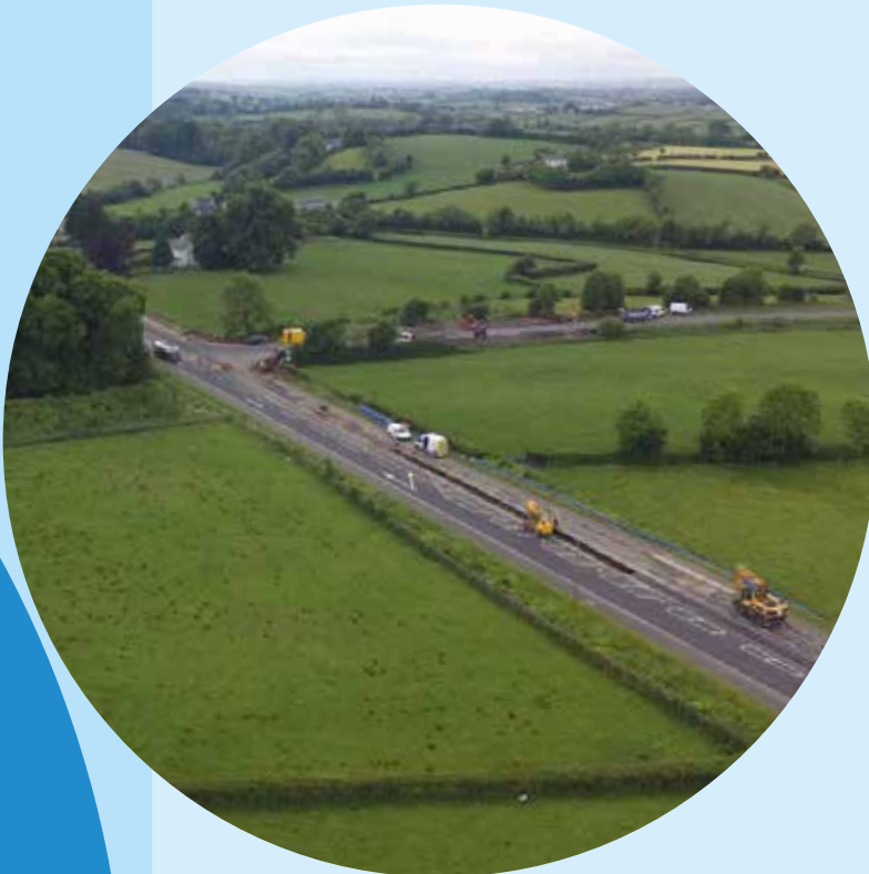
Aerial view of the Carland to Cookstown Trunk Main under construction.
