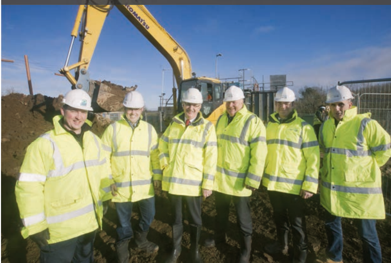
NI Water staff, contractor staff and Minister Kennedy pictured on site at Annacloy WwTW.
