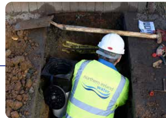
NI Water staff repairing supply interruptions
