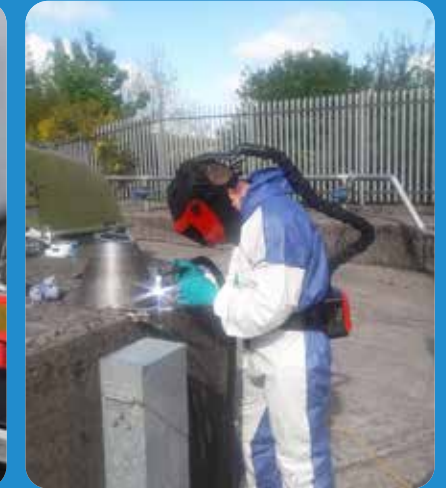
Mechanical and electrical operative repairing a screen
