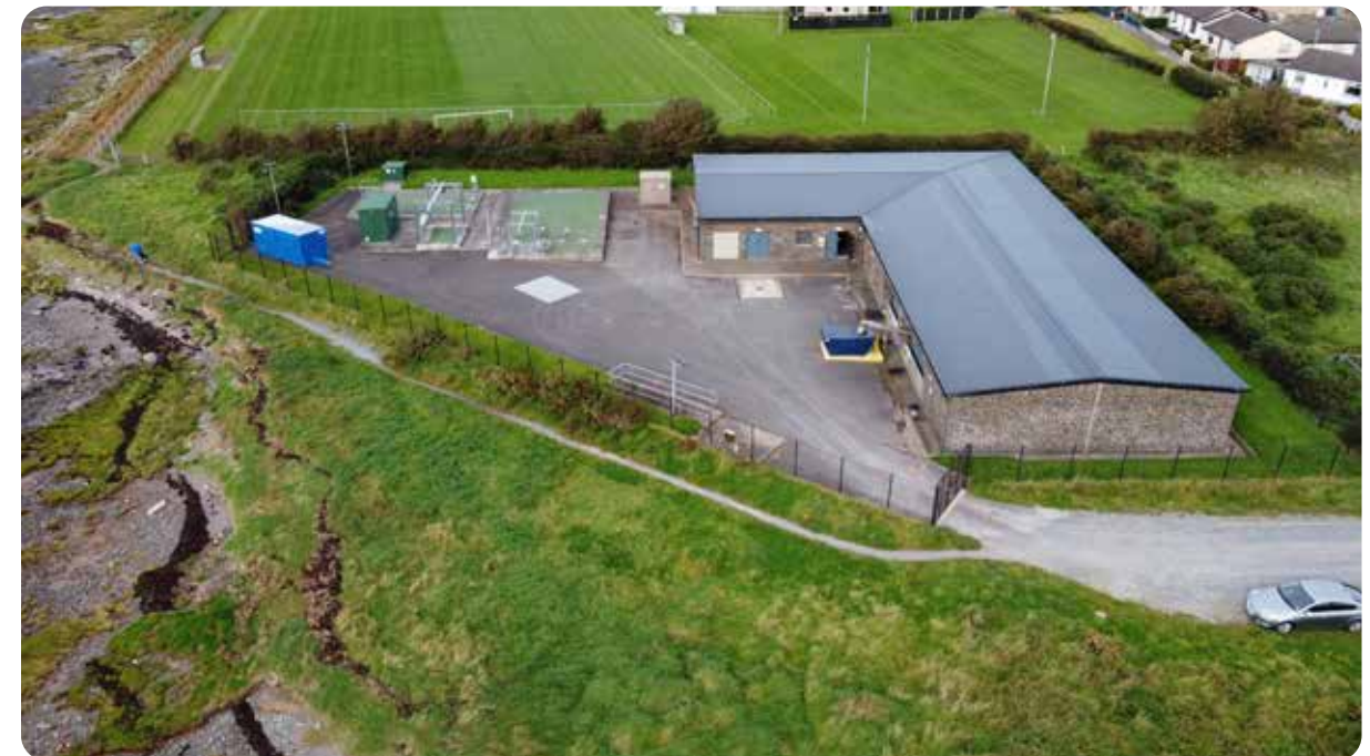
Greyabbey wastewater treatment works, County Down
