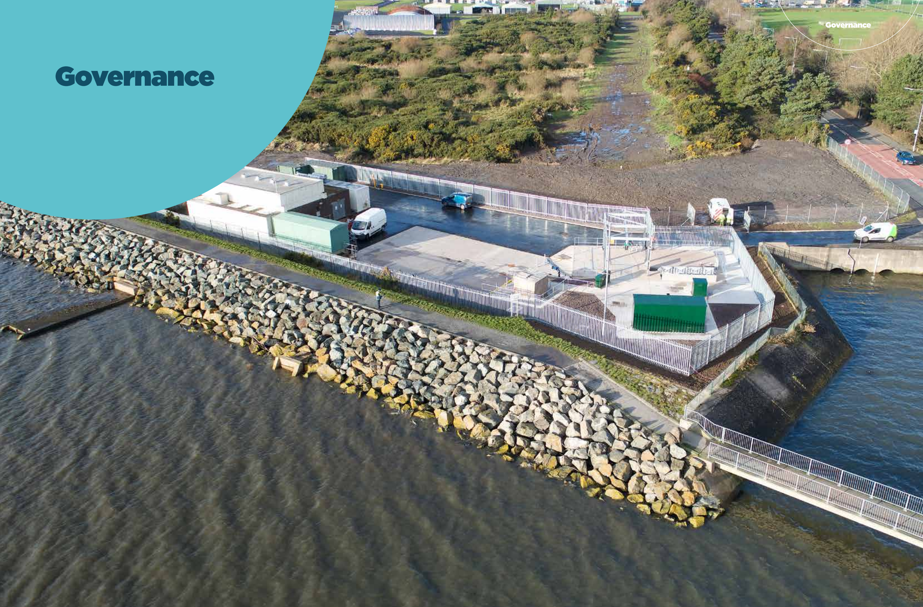
Portaferry Road wastewater pumping station, County Down
