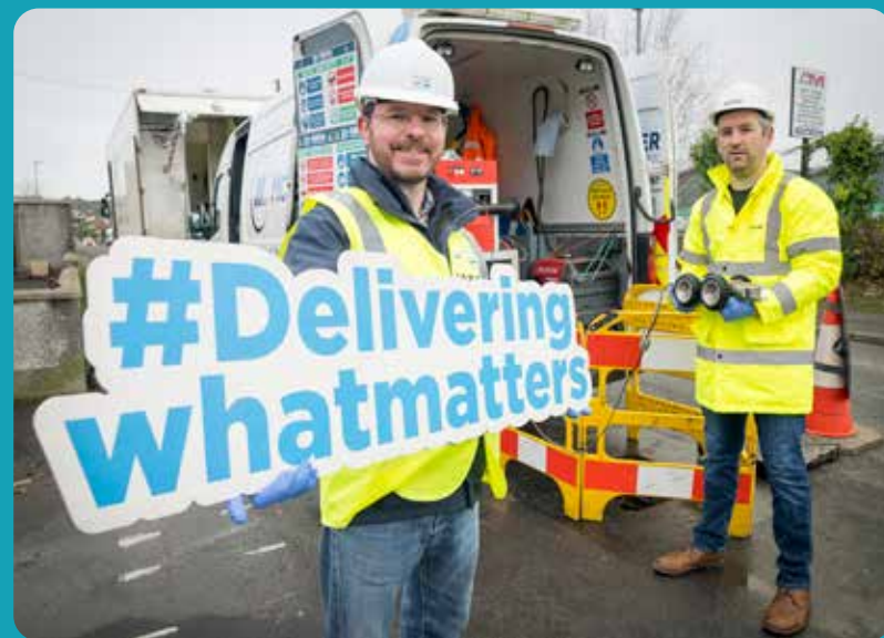
Sewer relining technology being used in wider West and South Belfast
