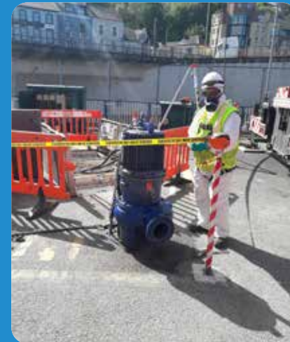
Submersible pump removal from 11 metre wet well at a wastewater pumping station
