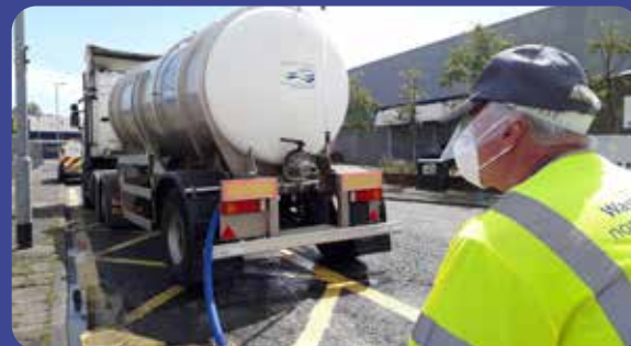
Tankering operations during the high demand event in May 2020
