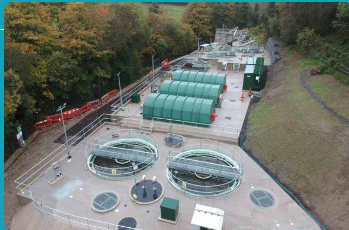
Completed SWELL wastewater treatment works at Donemana, County Tyrone
