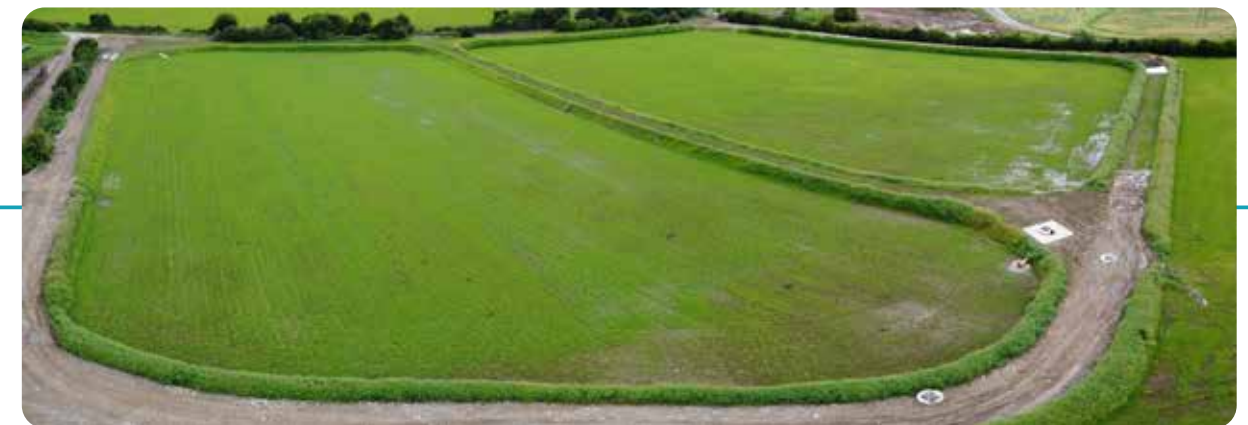
Ballykelly integrated constructed wetland, County Derry/Londonderry
