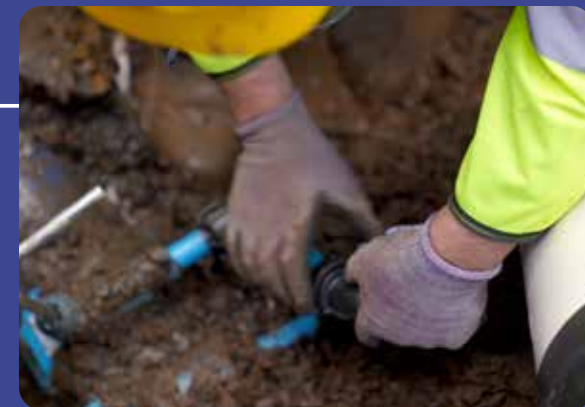
Repair to a burst pipe
