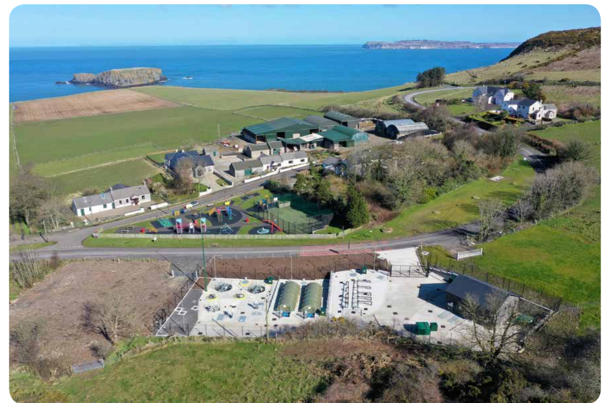
New wastewater treatment works under construction at Ballintoy, County Antrim
