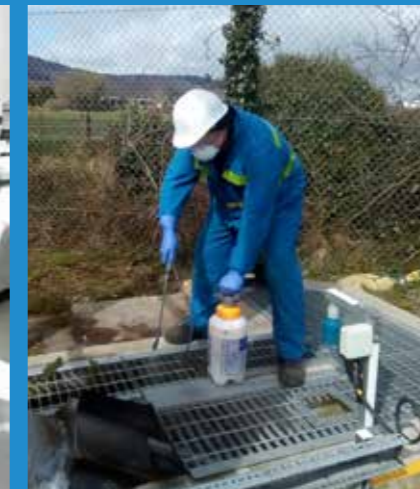
Mechanical and electrical craft fitter carrying out repairs
