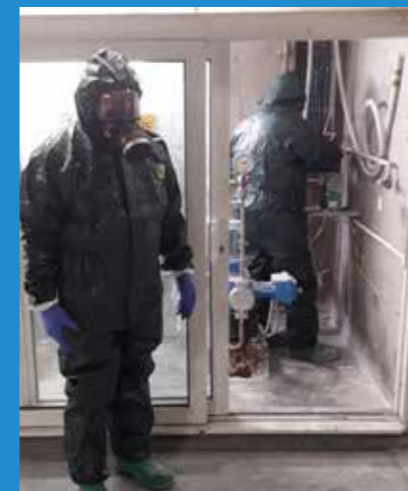
Water treatment operatives working on pumps
