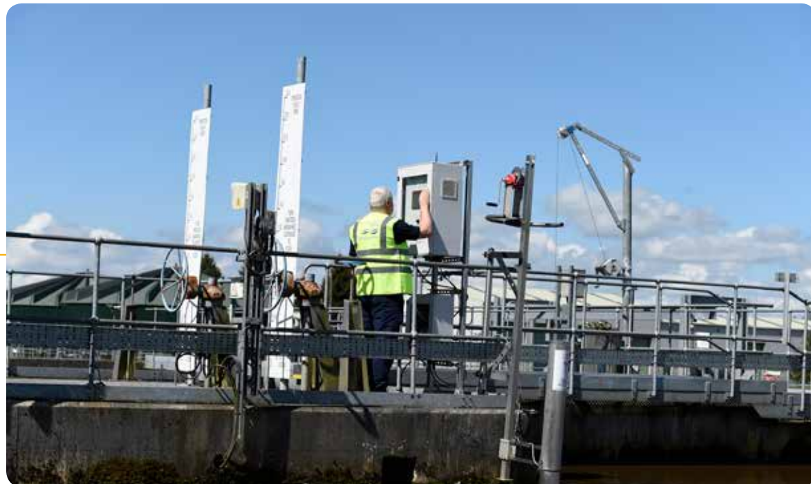
Antrim used water treatment works, County Antrim
