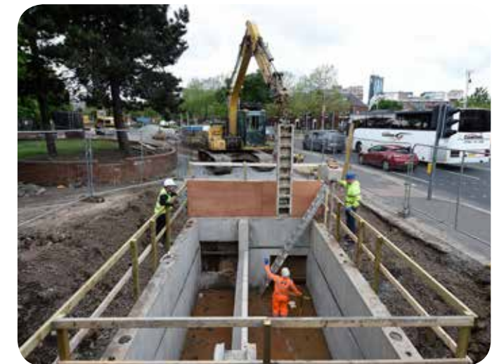
Storm water separation in Belfast city centre
