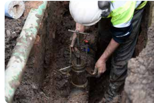
Lead communication pipes being replaced
