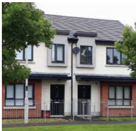
Social Housing at Deerfin/Derrycoole Way
