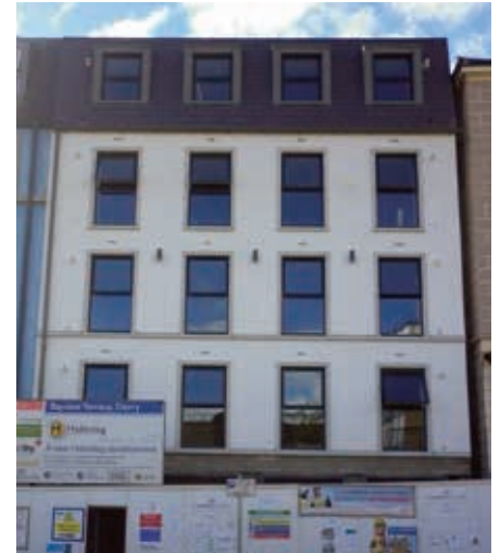
Social Housing Apartments under Construction at Bayview Terrace
