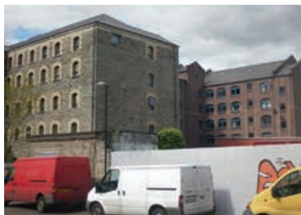
Re-improvement works at Rockmills
