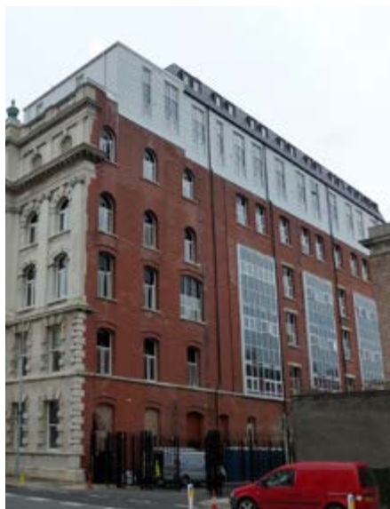
Purpose built student housing in Belfast
