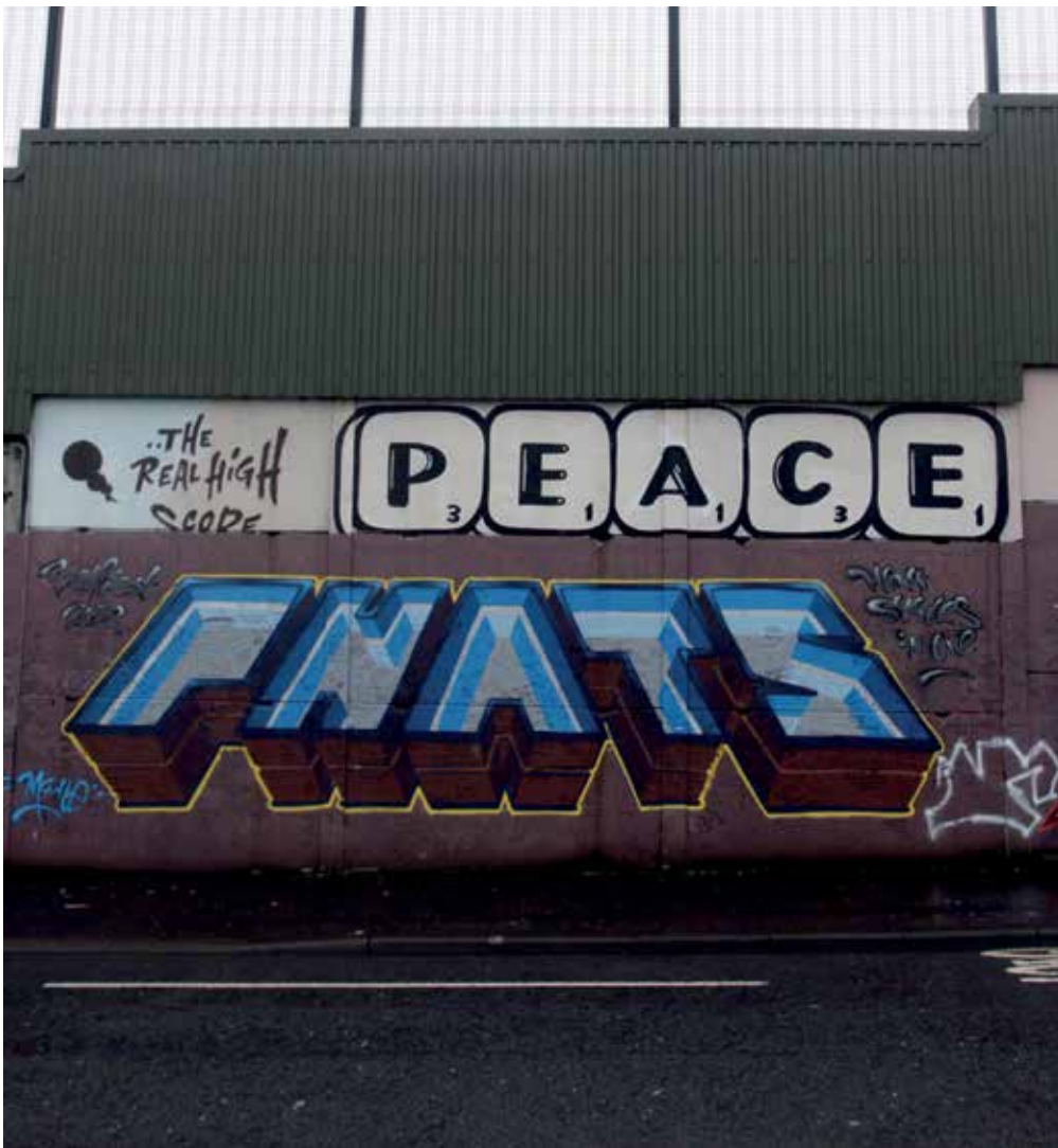
LEFT: The longest and tallest Peace Wall in Northern Ireland is at Cupar Way, Belfast. The multi-level barrier is 800 metres long and consists of a 4.5 metre high concrete wall, topped with 3 metre high metal sheeting and 6 metres of open mesh fence.
