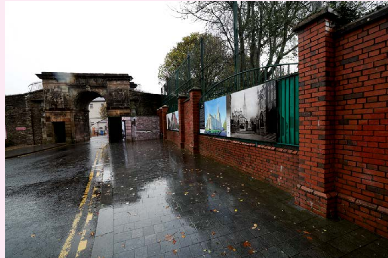
ABOVE: Bishops Gate interface in Derry/ Londonderry.
