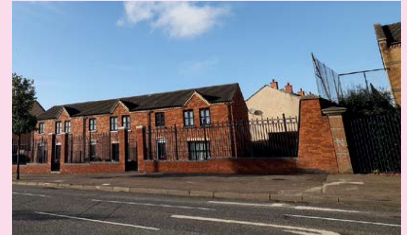
RIGHT: The transformation of a harsh Peace Wall on North Queen Street in Belfast has improved residents lives. They now have gardens and can access their house via the front door.
