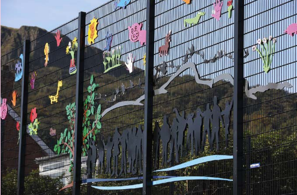
BELOW LEFT: The barrier on Flax Street, Crumlin Road, which has stood for more than 30 years.
