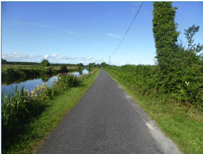
North towpath, view west
