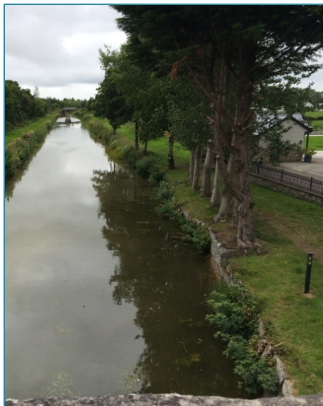
View from Colgans Bridge west to Georges Bridge
