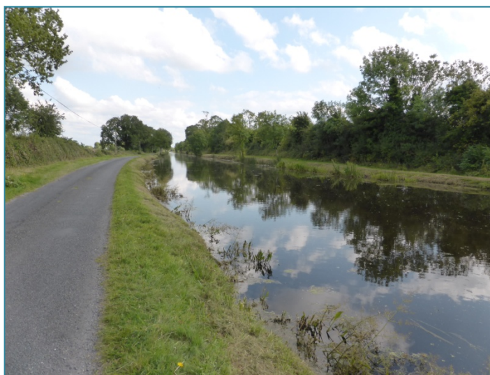
North towpath, view east
