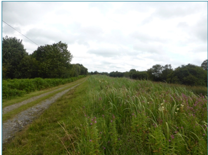
North towpath, view east
