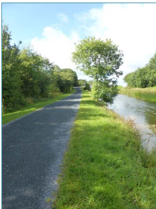
South towpath, view west
