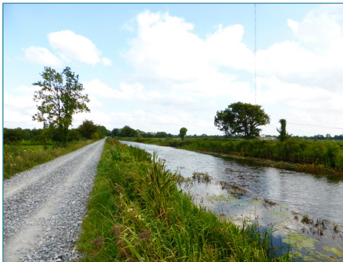
North towpath, view east
