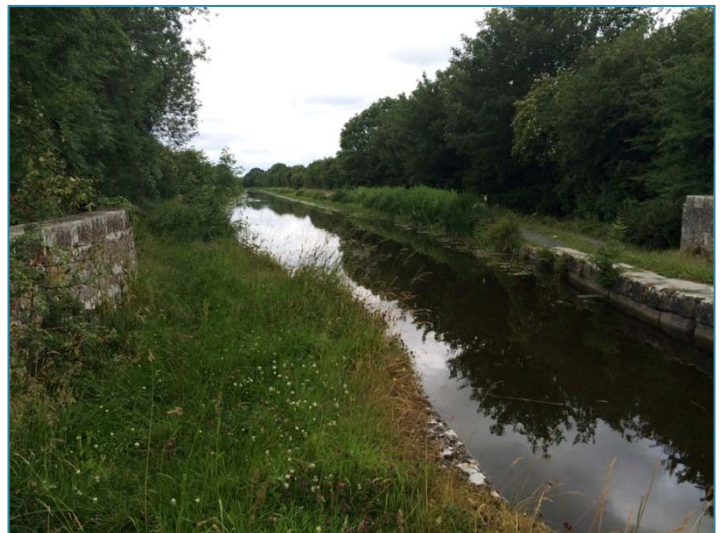
Huband Aqueduct, view east
