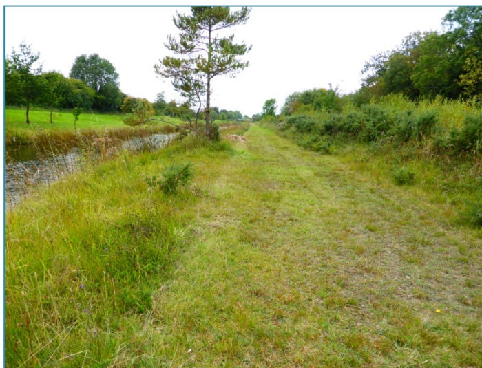
North towpath, view west
