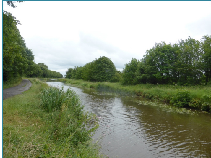
North towpath, view east
