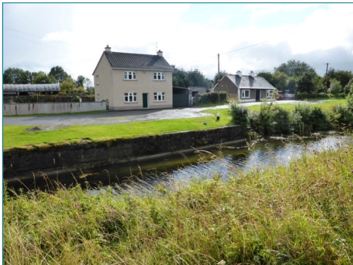
West of Armstrong Bridge
