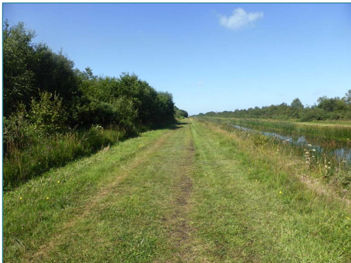
South towpath, view west
