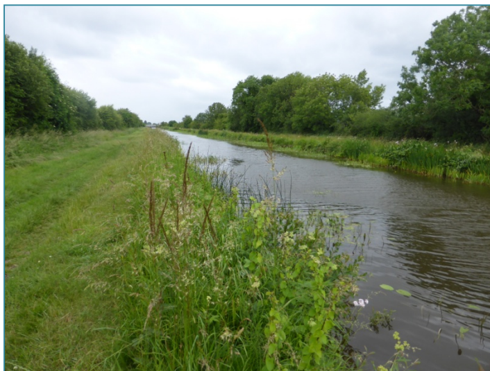
South towpath, view west
