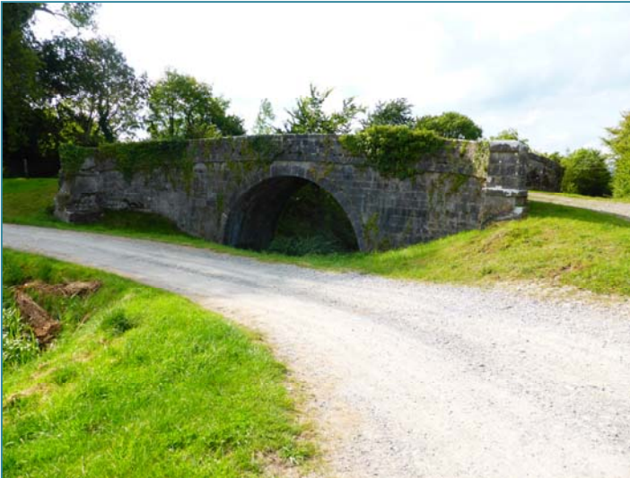
North towpath, Campbells Bridge
