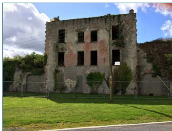
Shannon Harbour buildings
