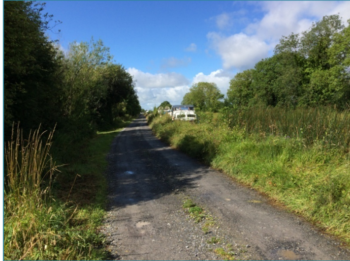
South towpath, view west
