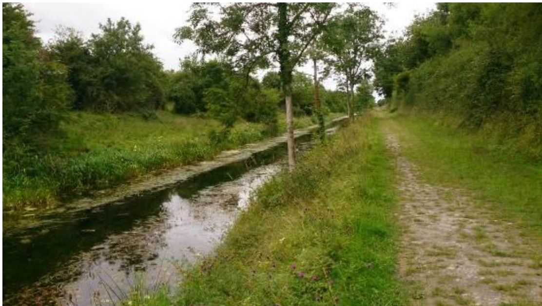
Plate 5.4 ESA4 on both sides of the canal
