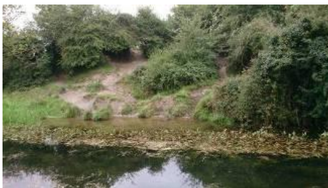
Plate 4.13 Canal bank between Burgh Bridge and 18 th Lock showing strong evidence of cattle poaching the banks
