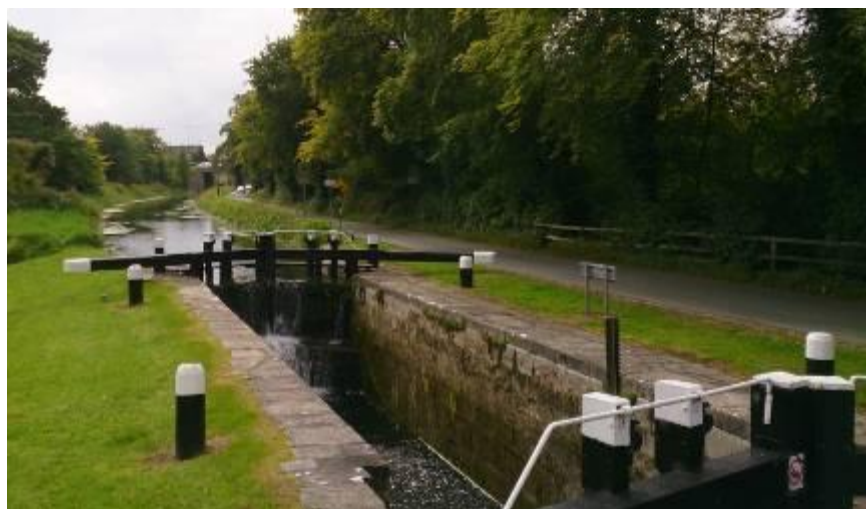
Plate 3.2 A section of the Grand Canal Main Line with typical features associated with canals, i.e. a lock and a paved towpath (now a road)
