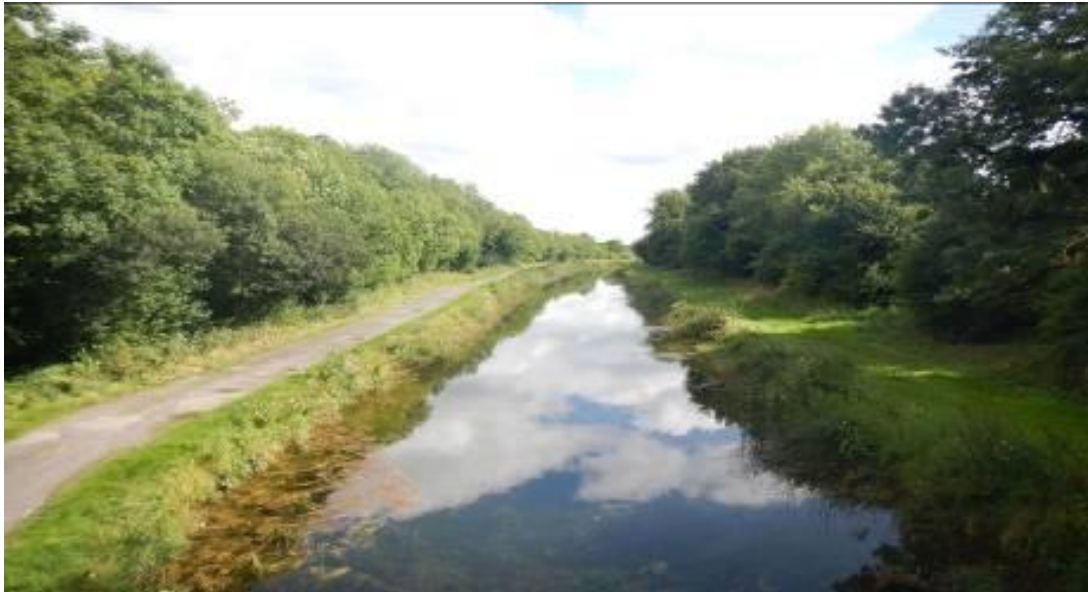
Plate 3.1 Example of TM Towpath Mosaic with both paved and grassy towpath on Mainline Canal section near Allenwood, Co. Kildare
