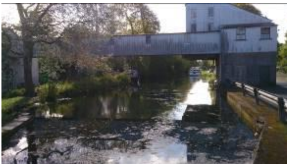
Plate 4.1 Area of BL3 at Leinster Mill
