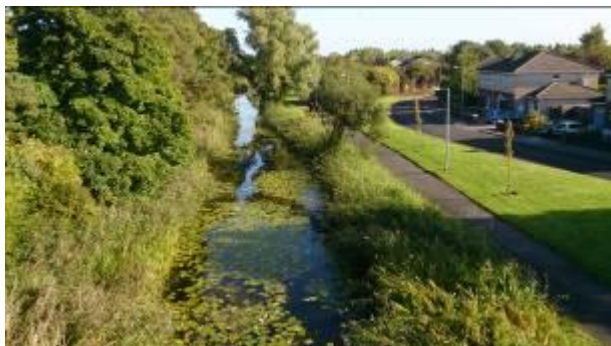
Plate 4.4 View northeast along the canal from Jigginstown Bridge
