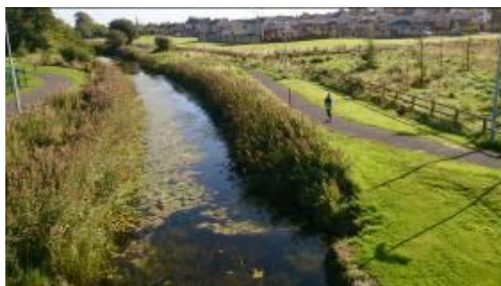
Plate 4.3 Section of canal on outskirts of Naas
