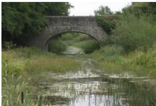
Plate 4.7.1 Diverse channel and emergent vegetation at Hoare's Bridge.
