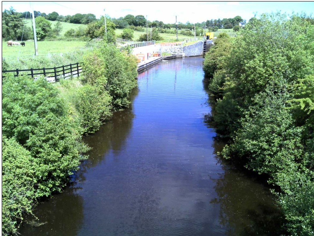
Plate 3.3. Canal section between Tiermactiernan Bridge and Lock 15
