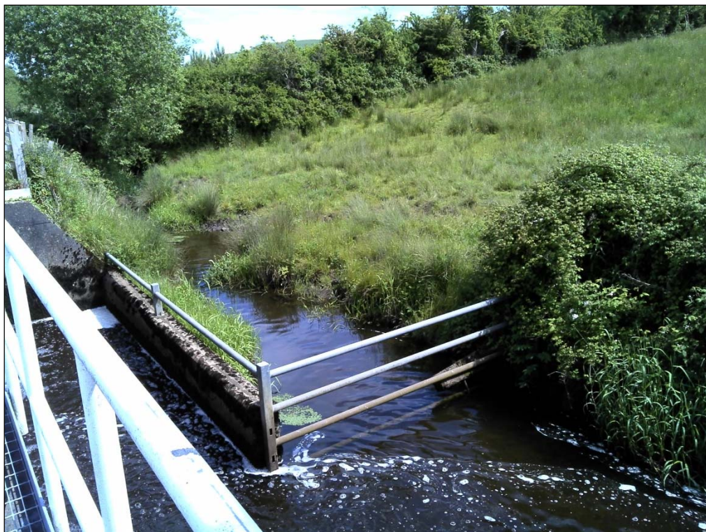
Plate 3.7. Drainage Ditch (FW4) on landward side of Towpath
