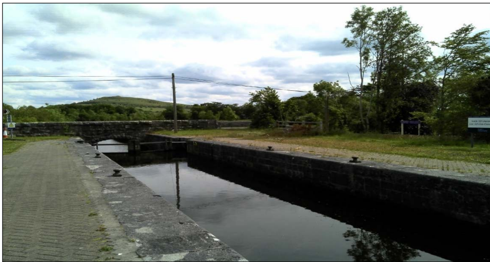
Plate 3.20. Example of Stone Walls and Other Stonework at Lock 12
