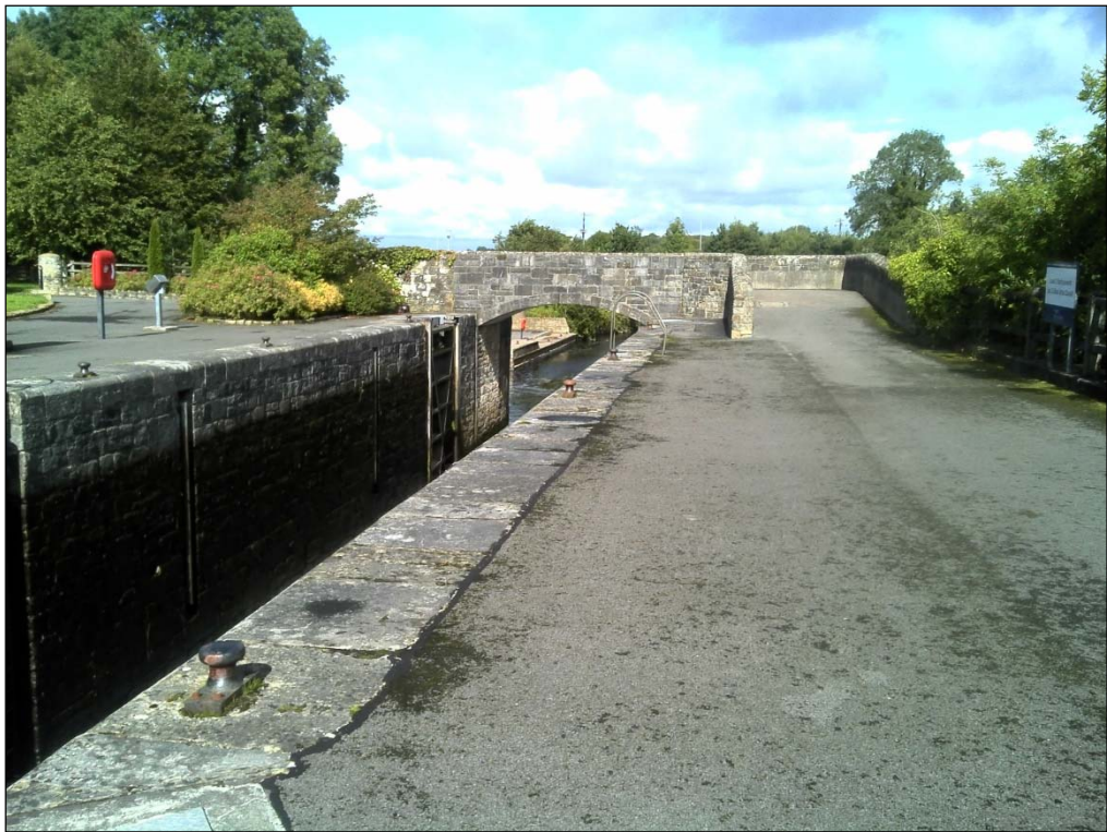
Plate 3.14. Example of Stone Walls and Other Stonework at Ballyconnell Lock 2
