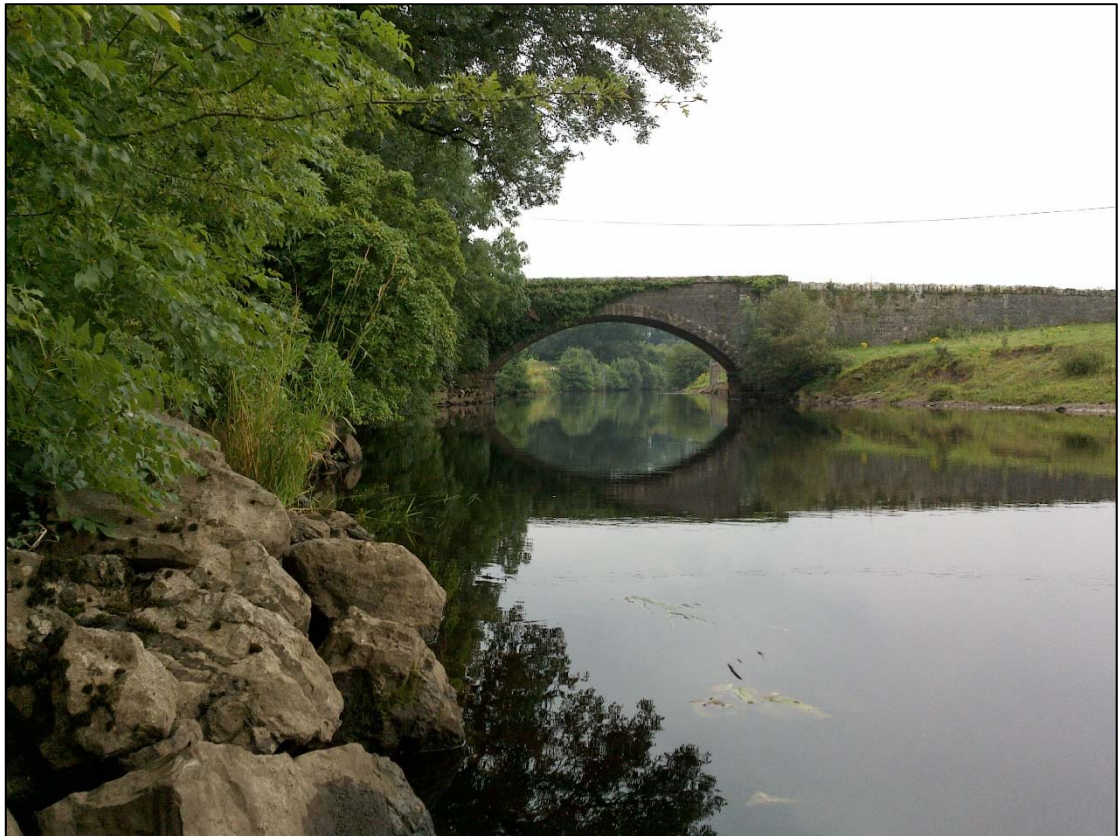
Plate 3.11 Example of Stone Walls and Other Stonework along Woodford River
