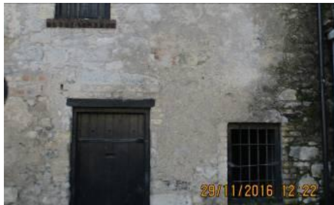
Photograph 5 View of remnants of original render
