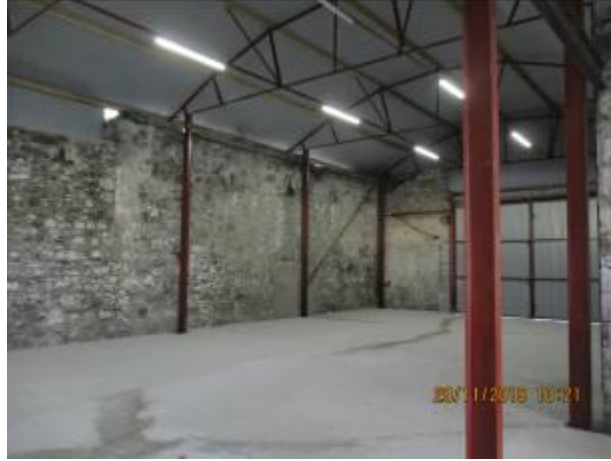
Photograph 4 View of interior of adjoining structure showing portal frame.
