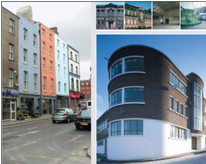
Photo 1 – Front Cover of Report Showing the Building Types
