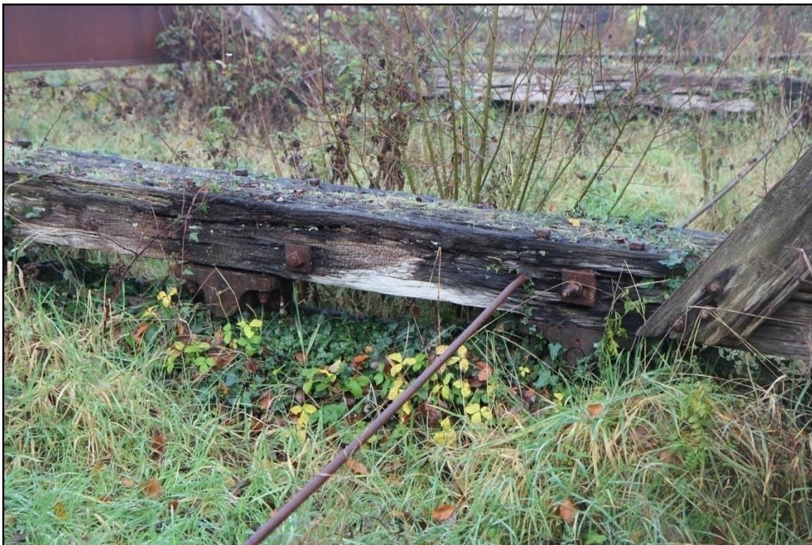
Photo 5 - Main Sliding Beam - Cast Iron Wheel/Runner
