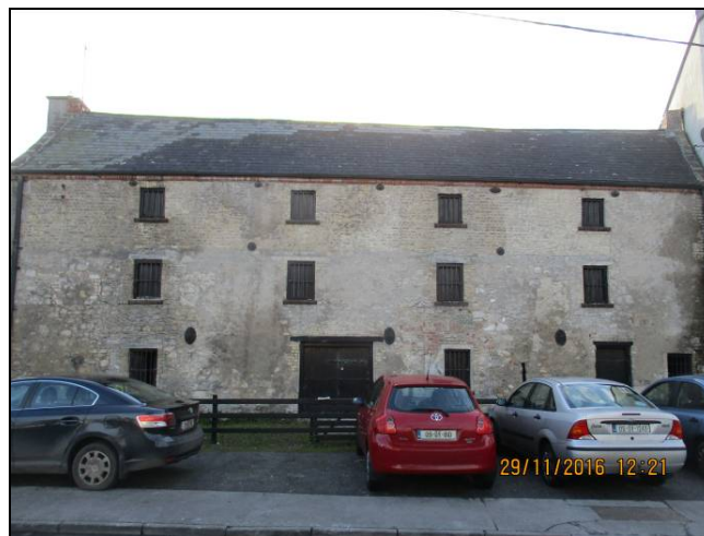
Photo 35 - Front roadside view of Young's Stores
