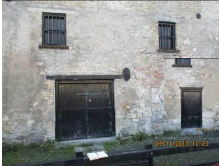
Photograph 8 View of external doors (main and inset)
