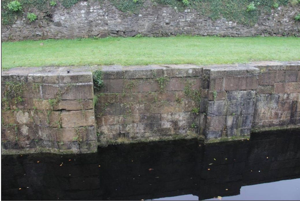
Photo 6 - The Old Lock Bridge
