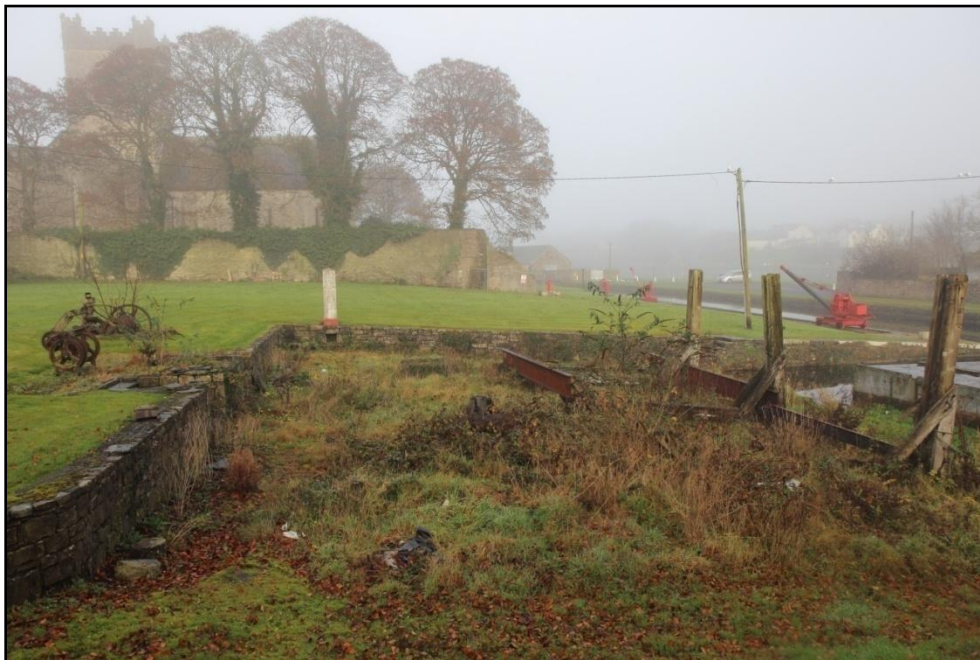
Photo 3 - Dry Dock/Slipway Area
