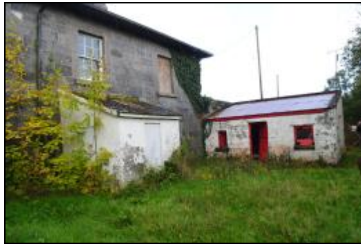
Photo 21 - Rear View of House and Sheds
