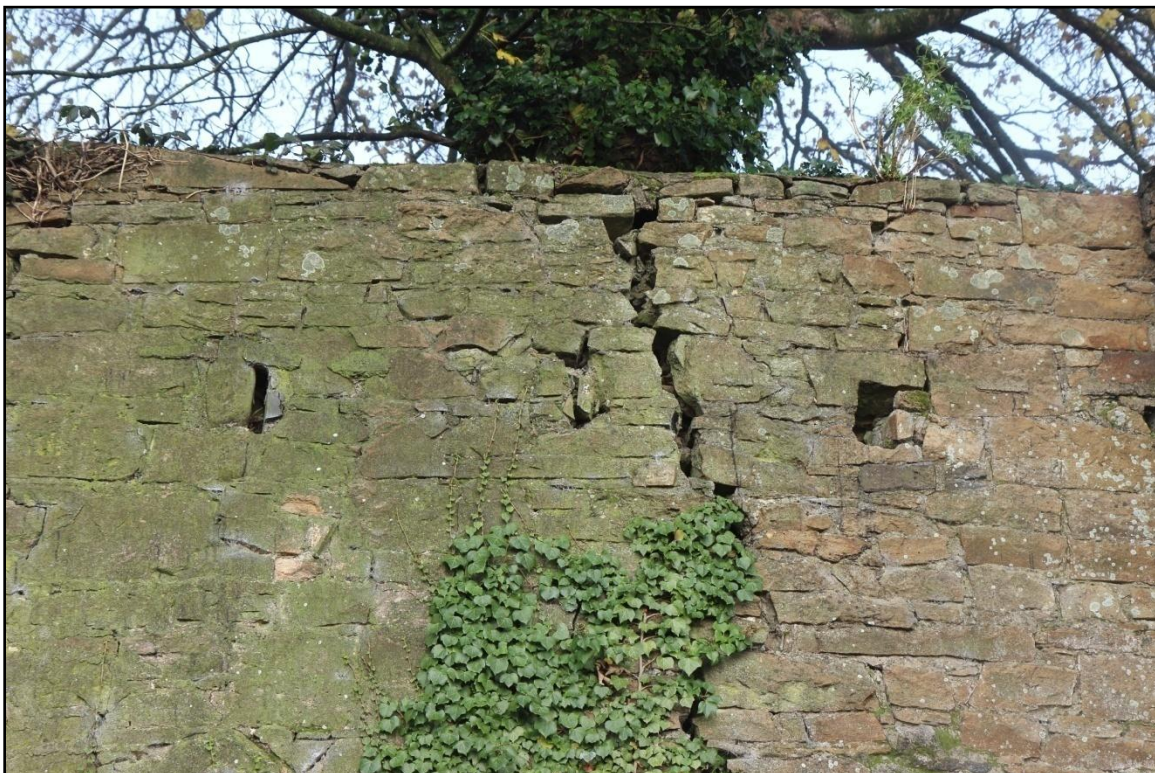
Photo 2 - Section of Cathedral Wall to be Monitored
