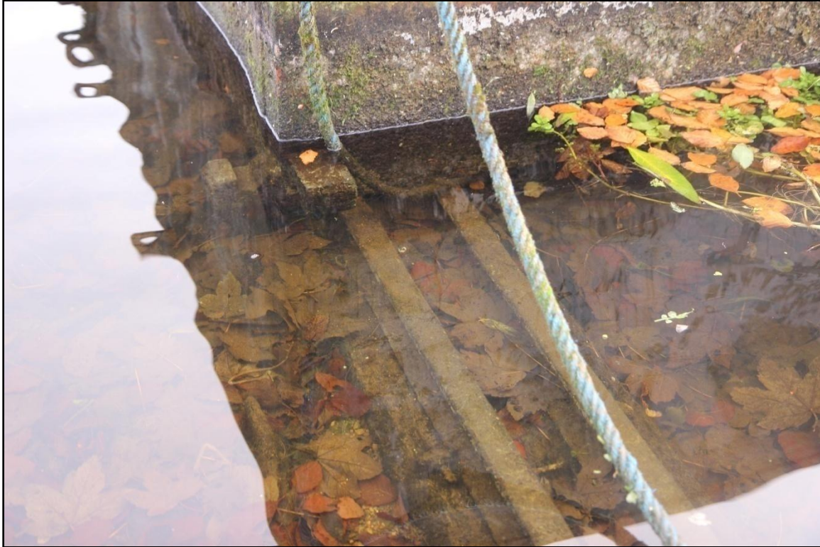
Photo 6 - Double Wrought Iron Track and Timber Base Entering Canal
