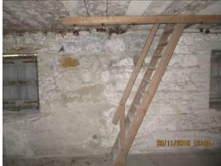
Photograph 6 View of interior wall (background), with “stair” access visible (foreground)
