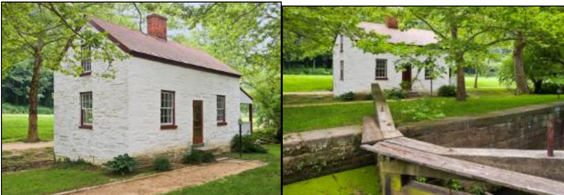
Photo 8 - Lockhouse 6 Sample Photos External
