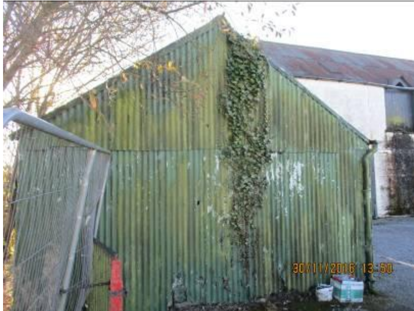
Photograph 9 View of gable end of corrugated iron shed with holes visible in the sheeting.
