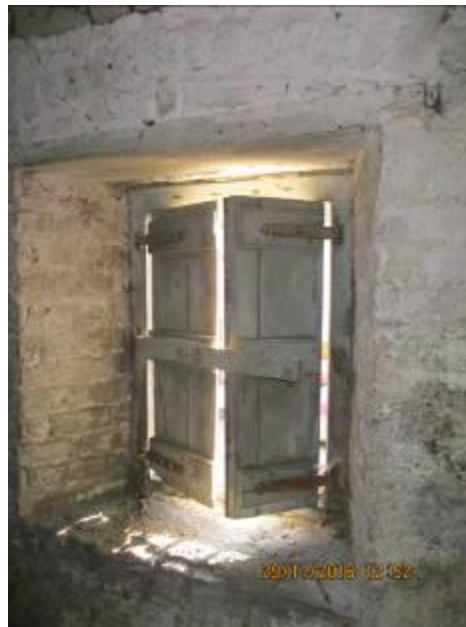
Photograph 7 Internal view of existing window assembly
