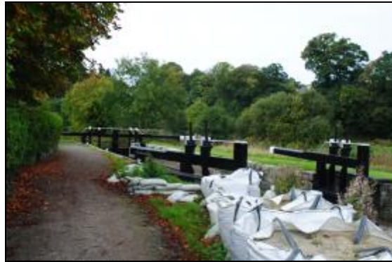
Photo 24 - Sandbags along the towpath at Lock 20
