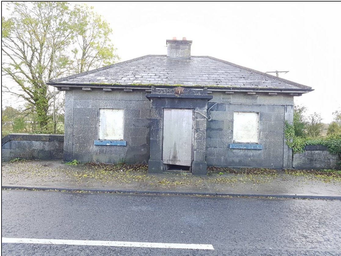
Photo 14 - Bridge Operator's House (Site Visit October 2016)
