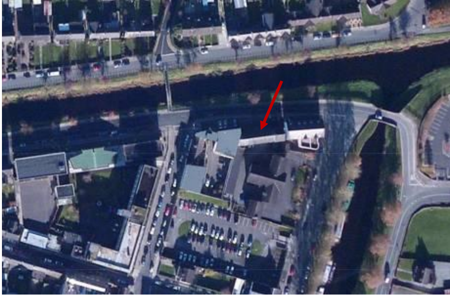
Figure 4 Ortho 2005 ©OSI License ACP Architectural Conservation Professionals AU 0067215
