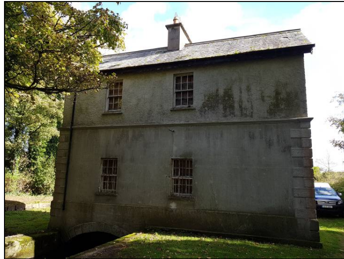
Photo 38 - Rear view of Lough Owel Sluice House from the Lake
