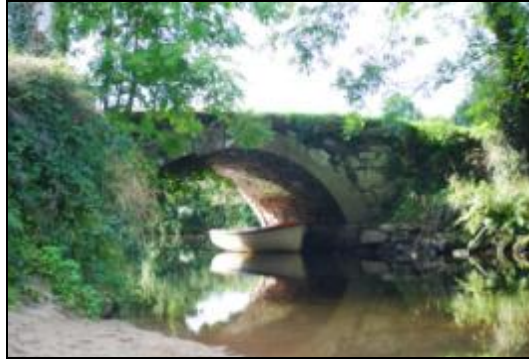
Photo 26 - Attractive Cut Stone Bridge Adjacent to House.
