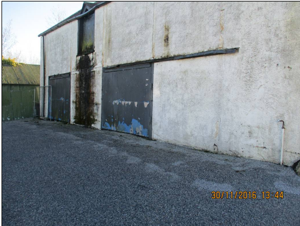
Photo 18 - Store House and Adjacent Galvanised Shed
