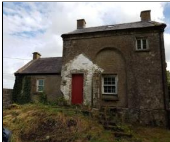
Photo 22 - Rear View of the Clondara Lock House
