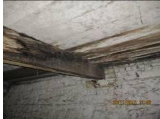
Photograph 2 Joist to First Floor
