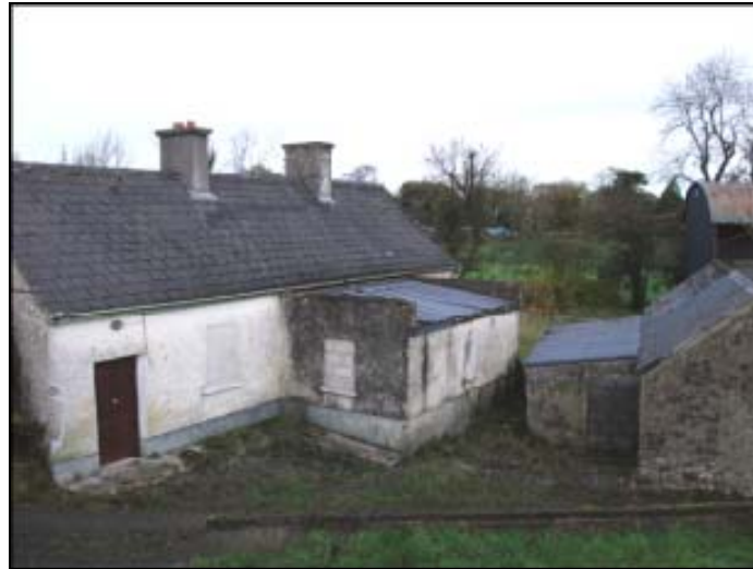
Photo 45 - House at Inny Aqueduct
