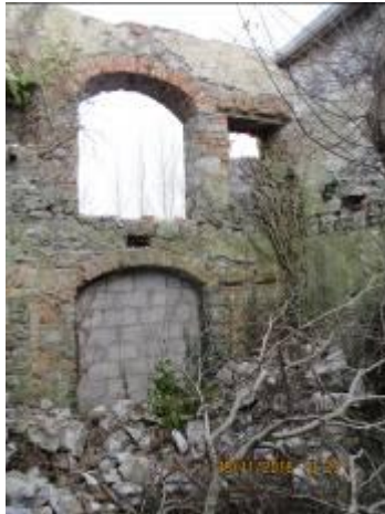
Photograph 1 View of interior of structure and vegetation growth.
