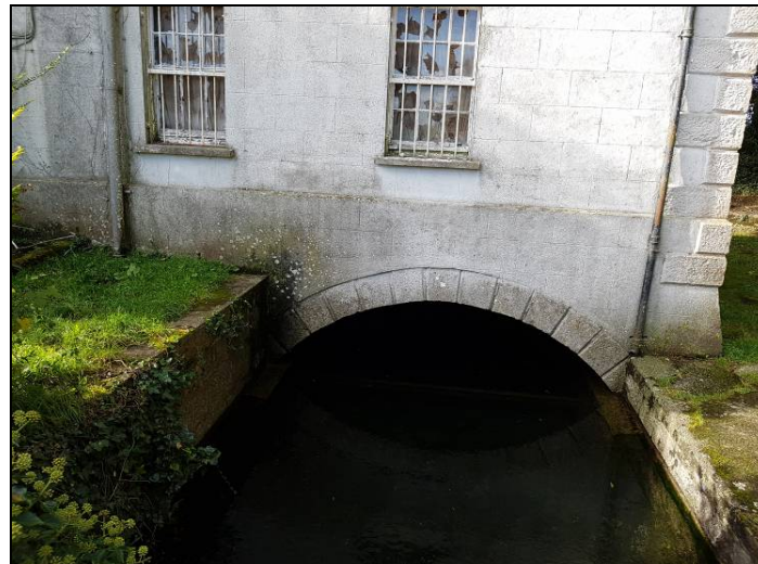
Photo 39 - Close up of Feeder for Canal Underneath the House.
