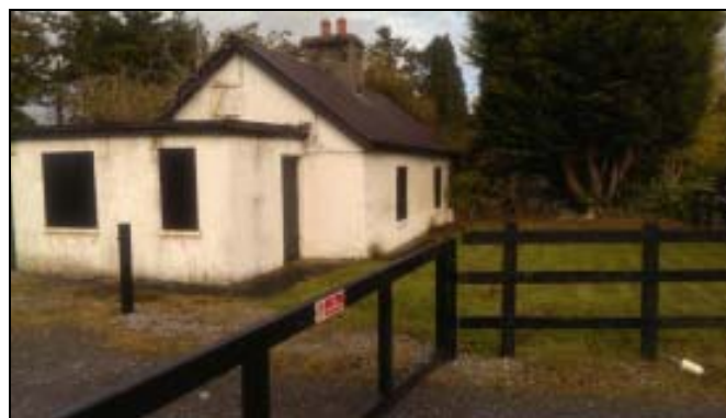
Photo 40 – View of Deey Bridge Lockhouse from Towpath
