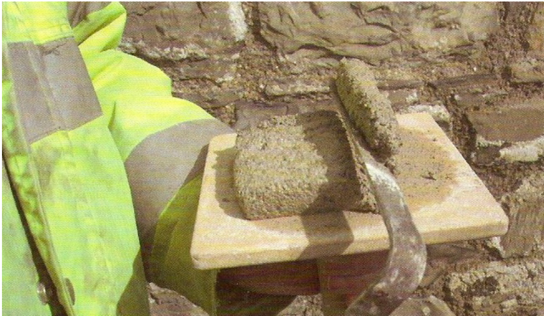
Pointing using pointing tool and small hawk
