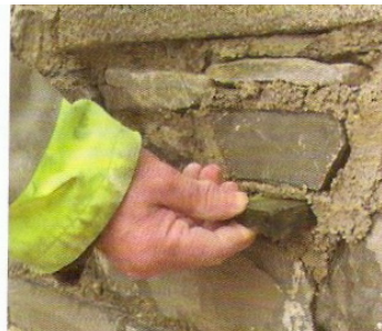
Inserting pinnings in large joints and tapping in
