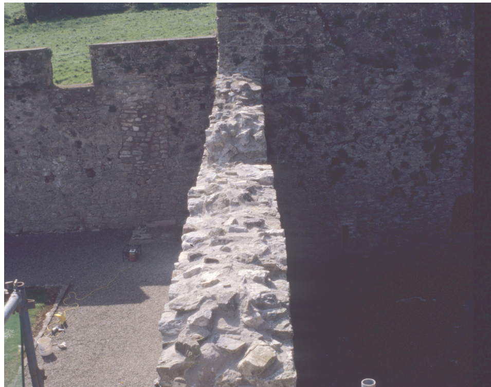
Rubble wall-top flaunched to allow water to run off as described at 7.9
