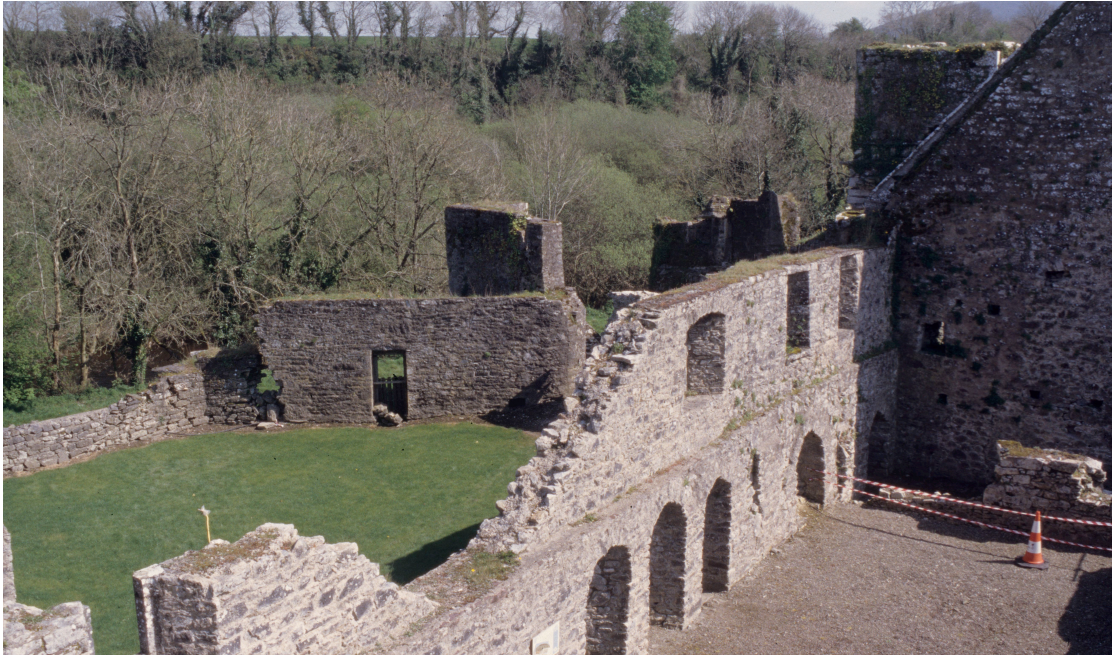
A well-maintained ruin where vegetation is controlled and wall tops are protected
