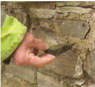
Inserting pinnings in large joints and tapping in
