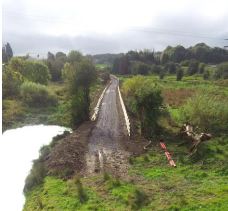
Figure 11: View of Monaghan greenway under construction.
