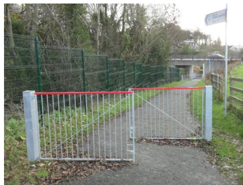
Figure 10: staggered gates prevent unauthorised vehicular access. The gates can be opened on request for events with large footfalls
