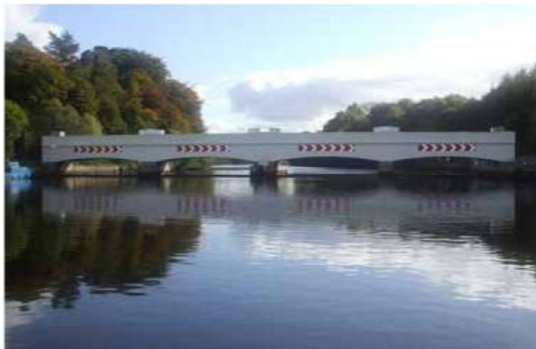
Bridge repair work
