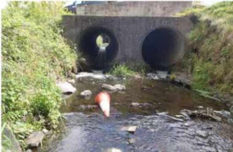
Culvert at Hillsborough
