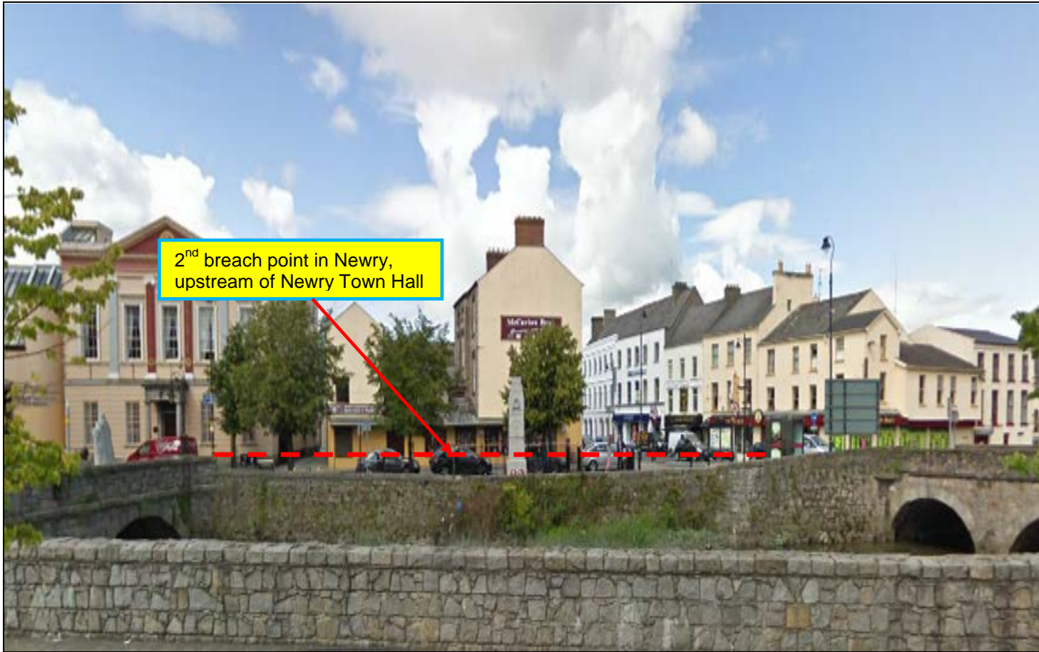
Photo 5.6.6.1 - Second breach point in Newry – Upstream of Newry Town Hall at the War Memorial
