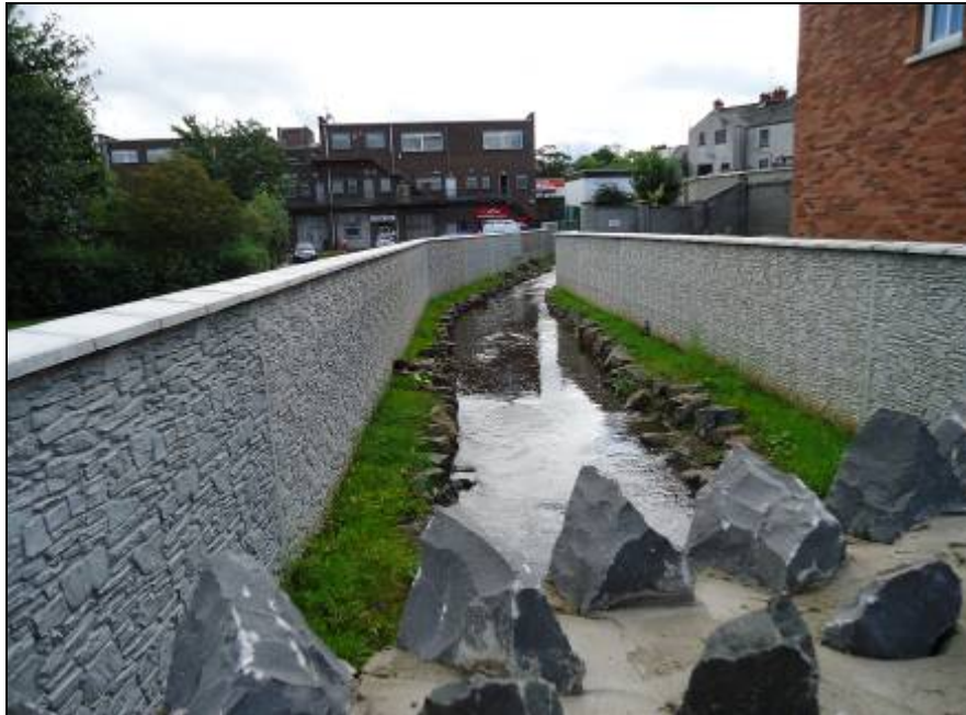
Photo 5.11.1.3 – New secant piled reinforced concrete flood wall with toe protection.
