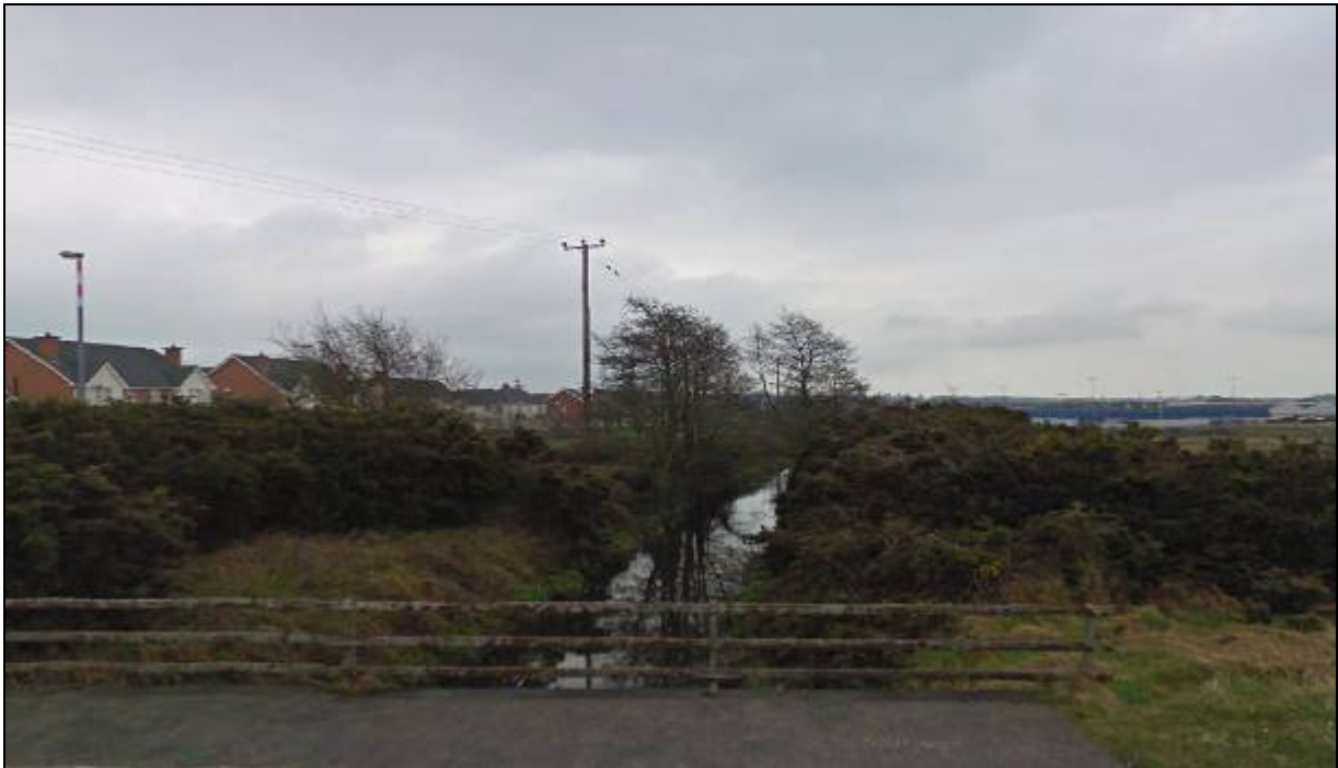
Figure 5.4.1.4 – Hollywell Burn Upstream, Antrim
