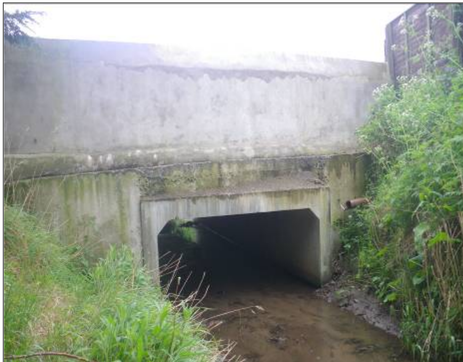
Photo 5.3.1.3 - Rivers Agency upgraded accommodation bridge on the Tirsogue Drain in Shanes Park, Lurgan
