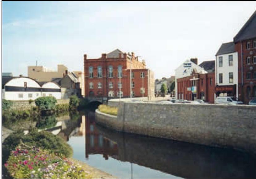
Photo 5.6.1.3 - Flood walls in Newry city centre after construction in 2003
