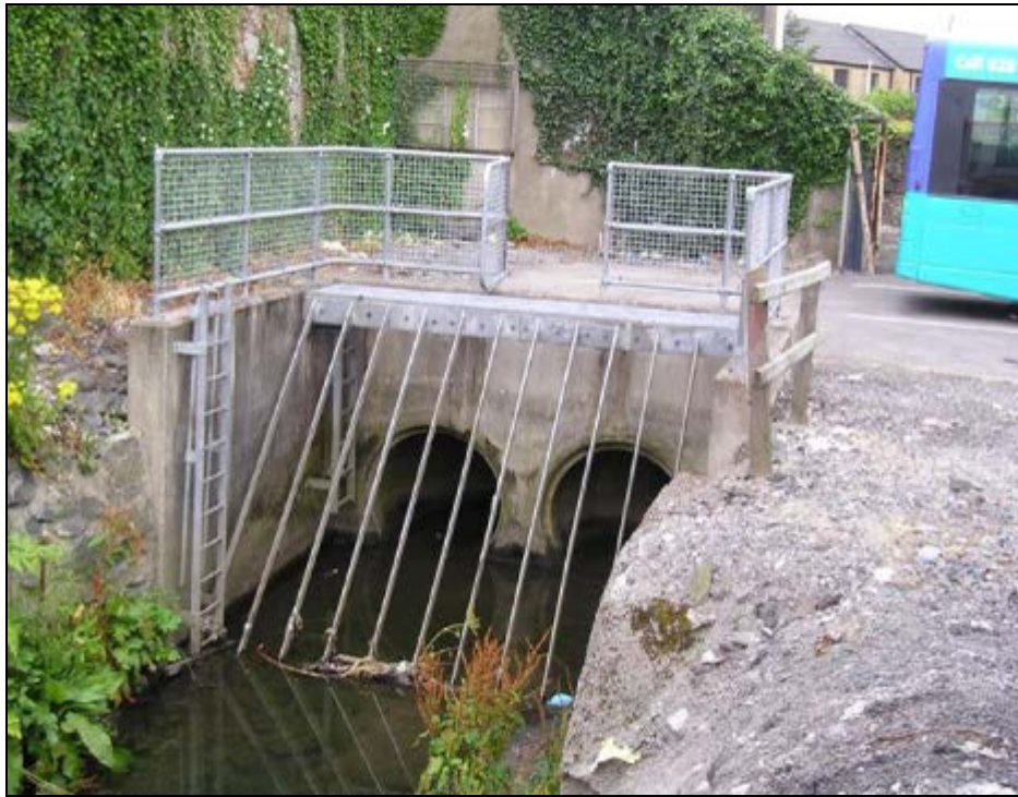
Photo 5.6.1.5 - Inlet Structure on Derrybeg River
