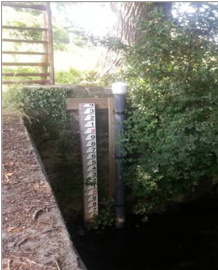
Photo 3.2.3 – Rivers Agency Text Alert Station
