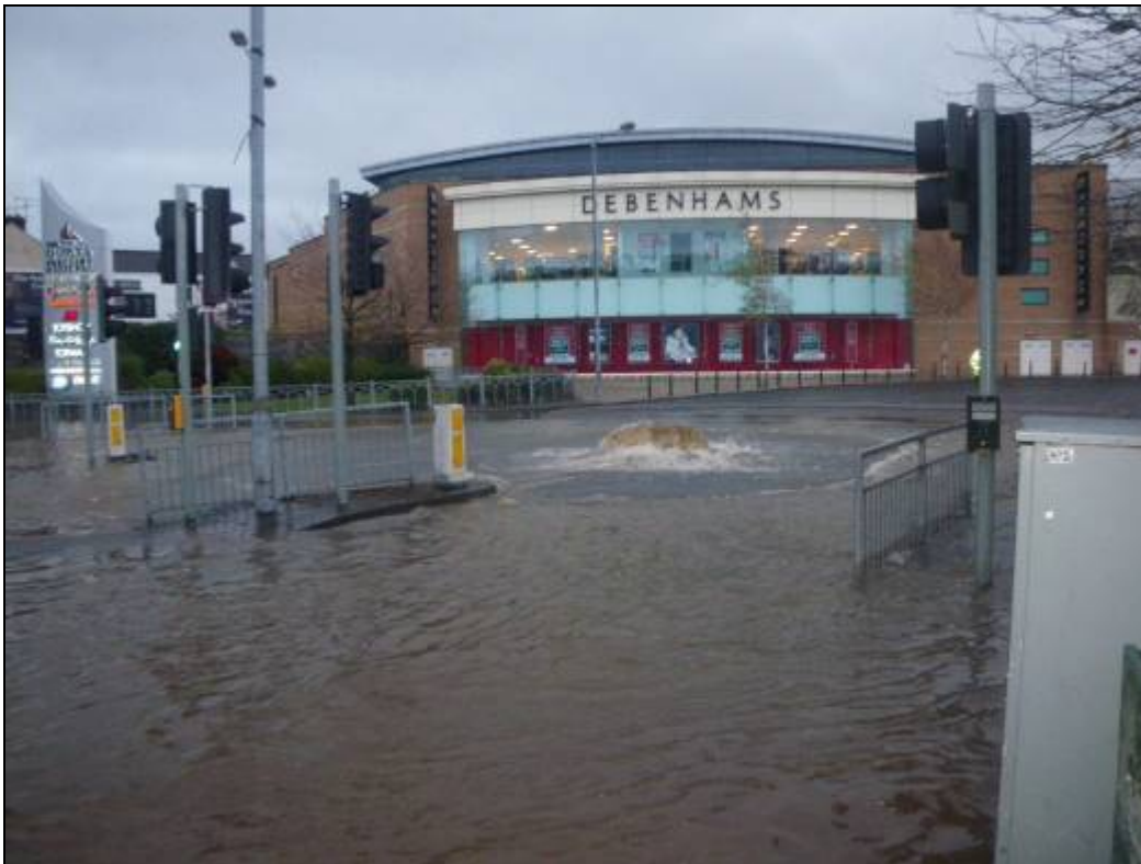
Photo 5.6.1.3 – N.I Water storm manhole surcharging, Newry 13 th Nov 2014
