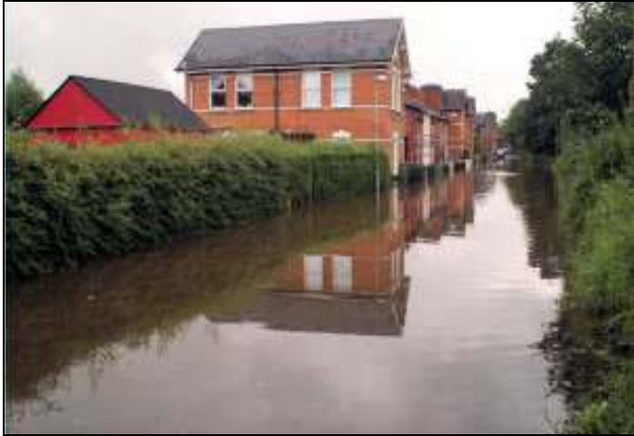
Photo 5.4.1.1 – Flooding at the entrance to Abbeyview 16 th August 2008.
