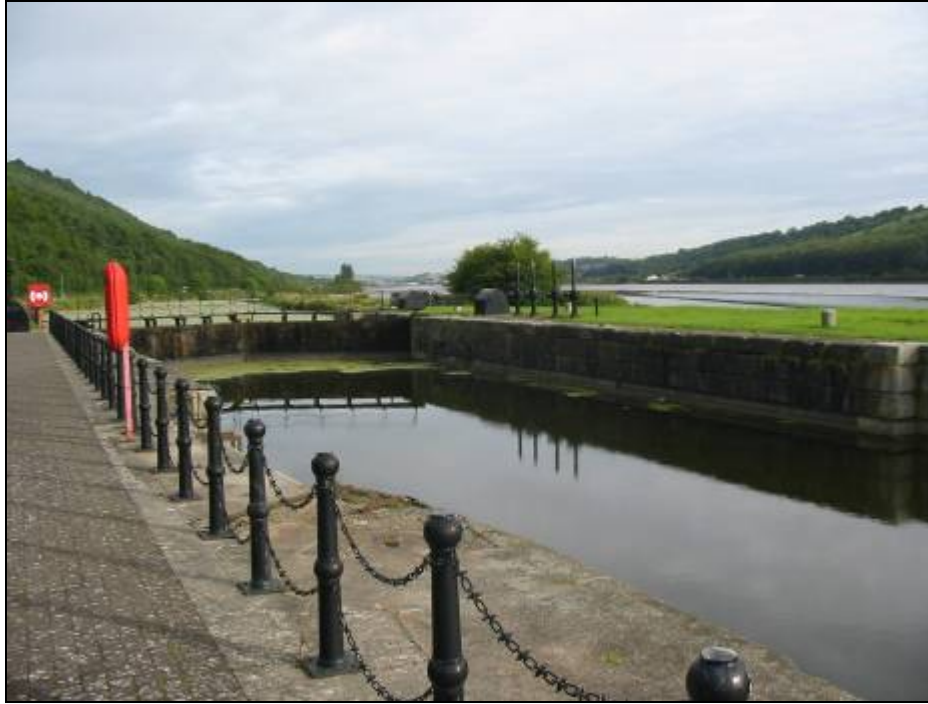
Photo 5.6.3.1 - Victoria Lock Gates on the Newry Canal
