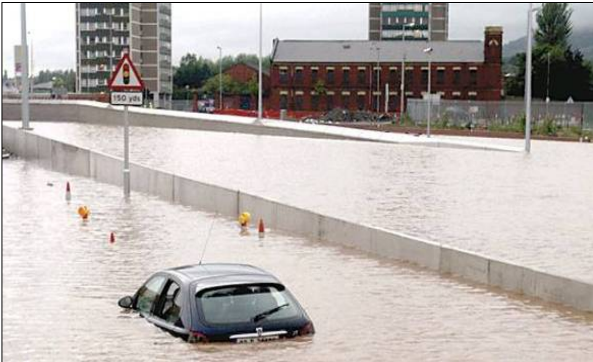
Photograph 5.3.1.2 - Flooding of West Link (Broadway Underpass), 16 August 2008
