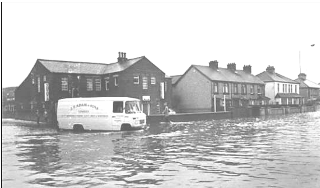
Photograph 5.8.1.1 - Flooding at Portaferry Road (Dec 1981)
