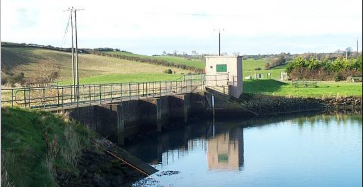
Photo 5.4.3.1 - Quoile Barrier (sea facing aspect)
