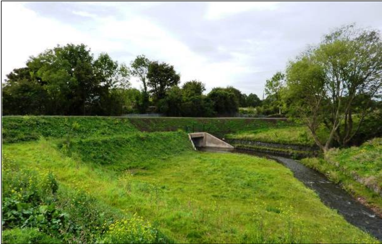
Photograph 5.9.1.1 – Sullatober Water Flood Alleviation Scheme (2014) – Culvert and Flood Storage
