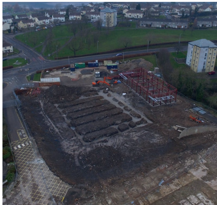
Work began on the new NIAS Enniskillen Station during 2016-17
