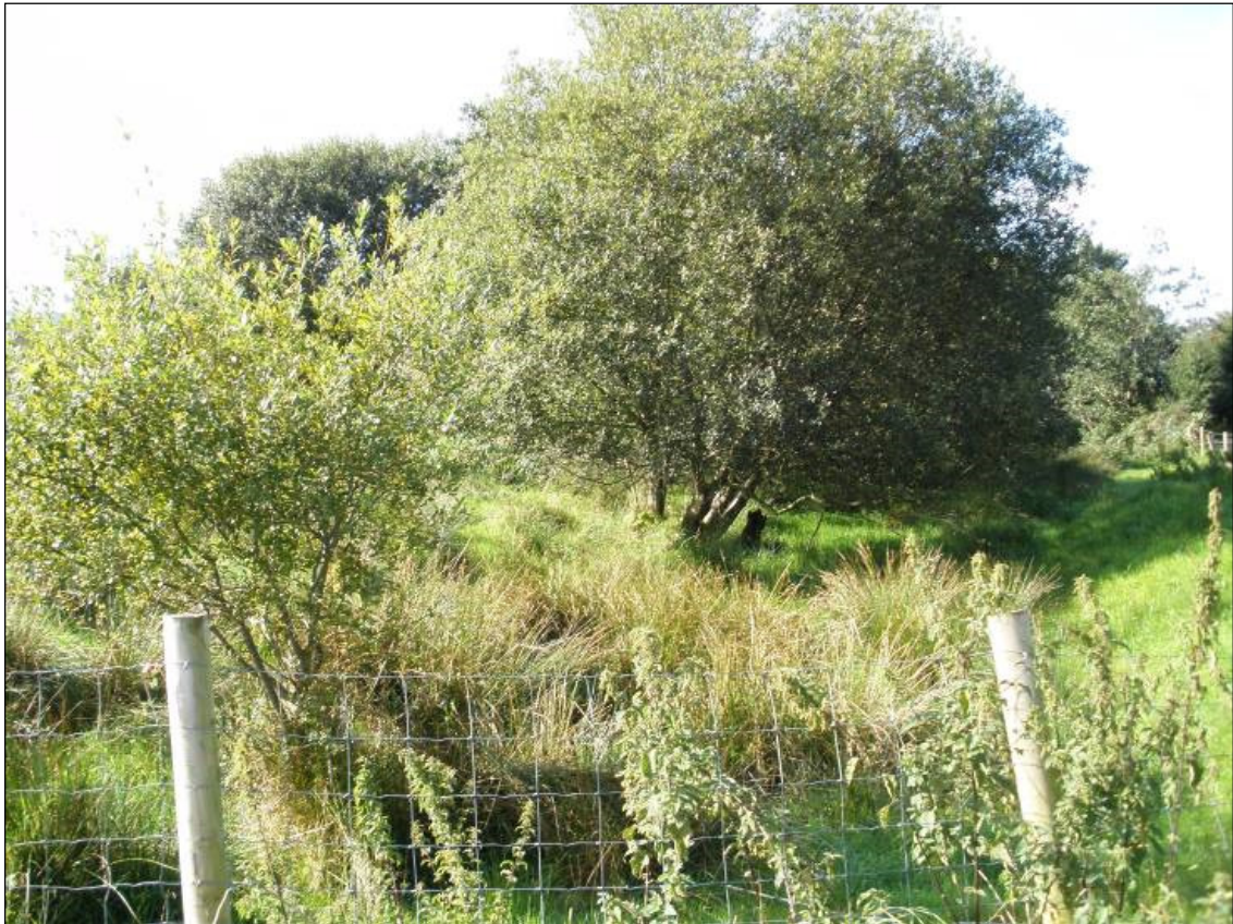
Plate 9.4 Strabane Canal in present overgrown state looking south west
