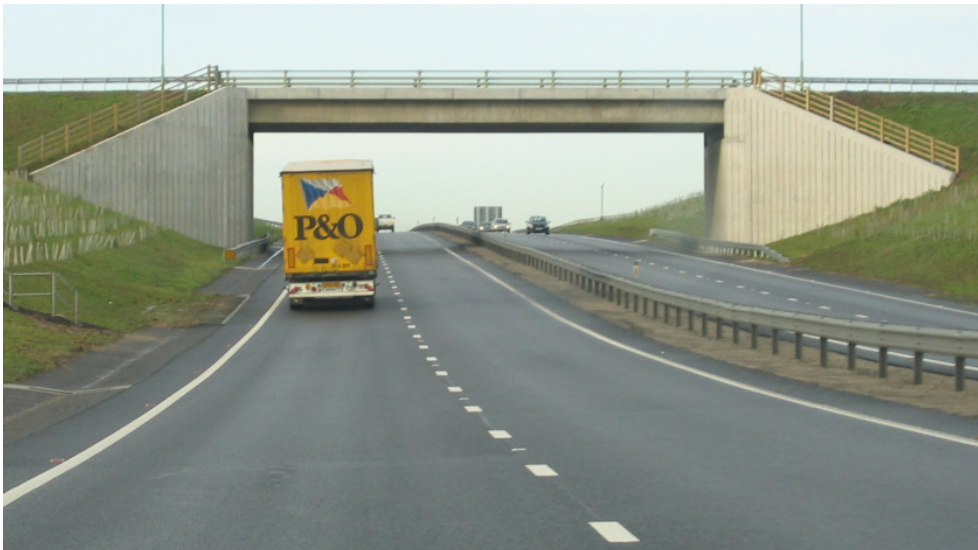
Plate 6.3 Typical single-span overbridge
