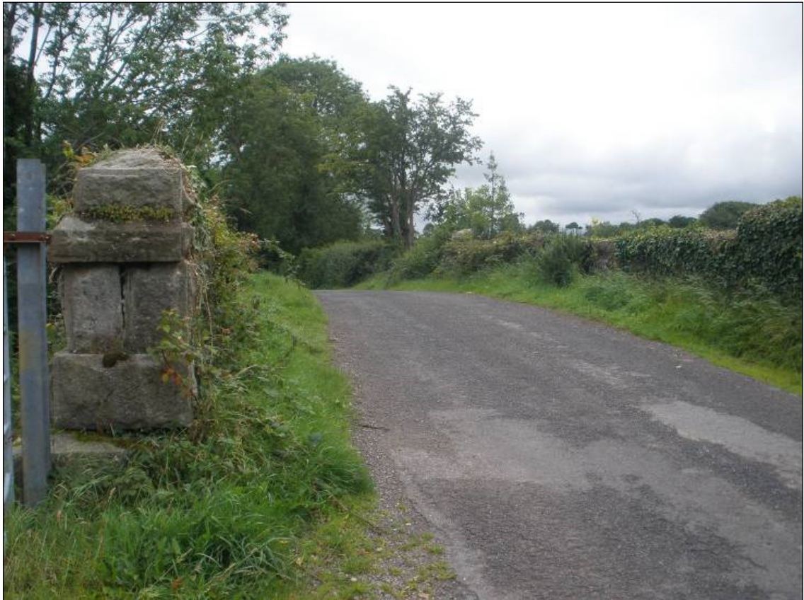
Plate 9.6 IHR Bridge Site 63 looking east
