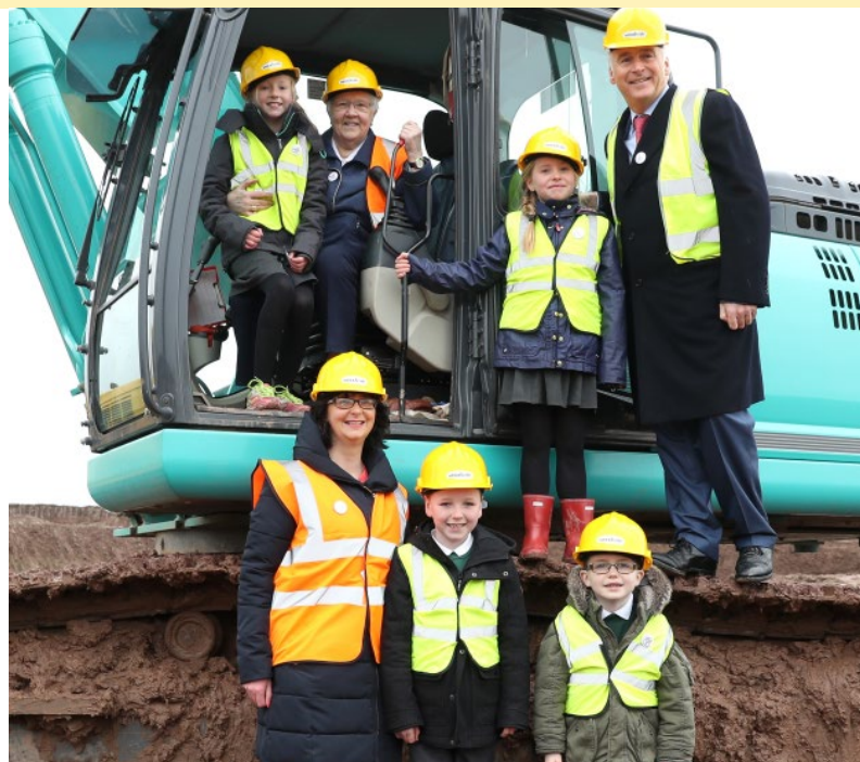
Baroness May Blood (in the driving seat!) with John Fitzpatrick (back, right), Acting Principal Siobhan Taggart and Omagh IPS pupils at the building site
