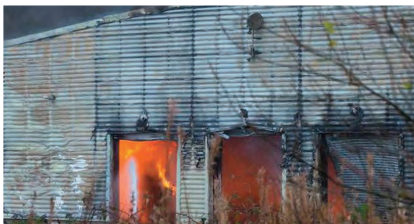
Major fire at Brickkiln Waste Management Facility
