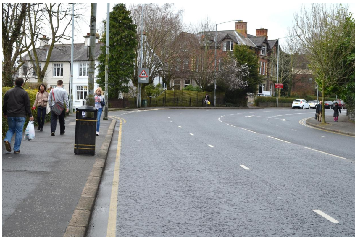
Figure 1: Approach to the Malone Road and Sans Souci Park junction
