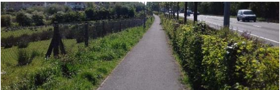
Photographs 32, 33 & 34: Offline Footway adjacent to the A5 Great Northern Link (See Drawing D-021 for all)
