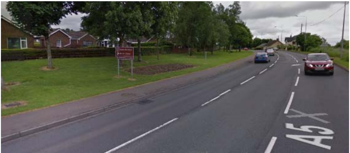
Photograph 25: A5 Victoria Road immediately north of the junction with Woodend Road (See Drawing D-007)
