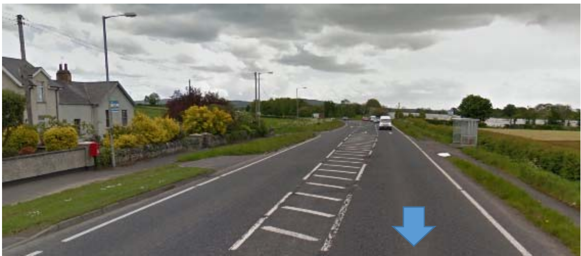
Photograph 7: Southbound on A5 Victoria Road, North of Willow Road (see drawing D-031)
