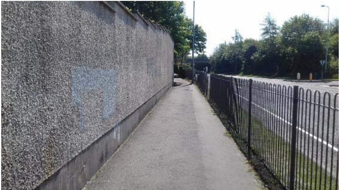
Photograph 36: Offline Footway adjacent to the A5 Great Northern Link (See Drawing D-021)
