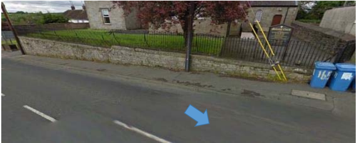
Photograph 7: Addition of Shared NMU facility (wall to be offset 1m) (See Drawing D-030)
