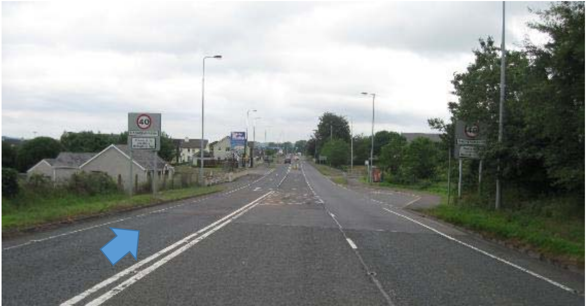
Photograph 6: Northbound entrance to Magheramason (See Drawing D-003)
