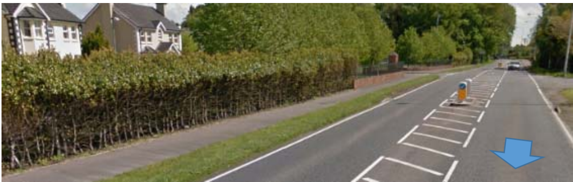
Photograph 1: Southbound footway of the A5 Beltany Road outside the Beltany Grove Residential Development (See Drawing D-019)
