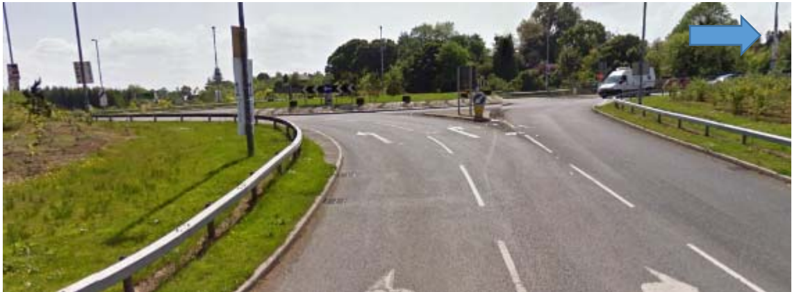
Photograph 14: Southbound on the A505 towards the Crevenagh Rd. Roundabout (See Drawing D-024)
