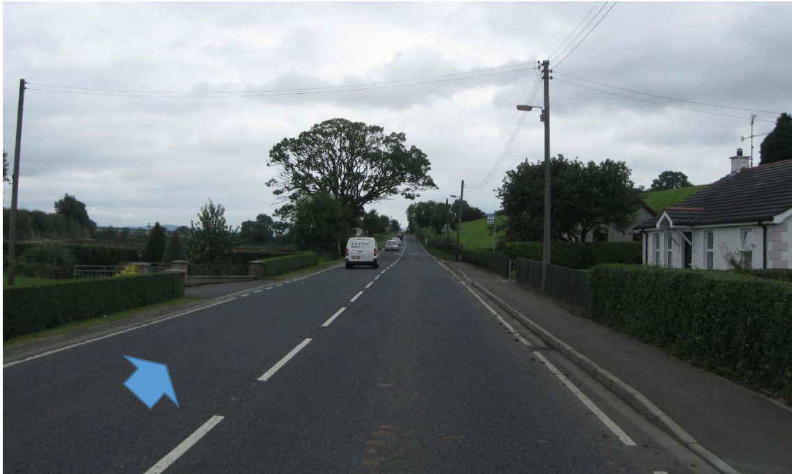
Photograph 5: Northbound on the A5 Victoria Road south of the Bready Reformed Presbyterian Church (See Drawing D-004)
