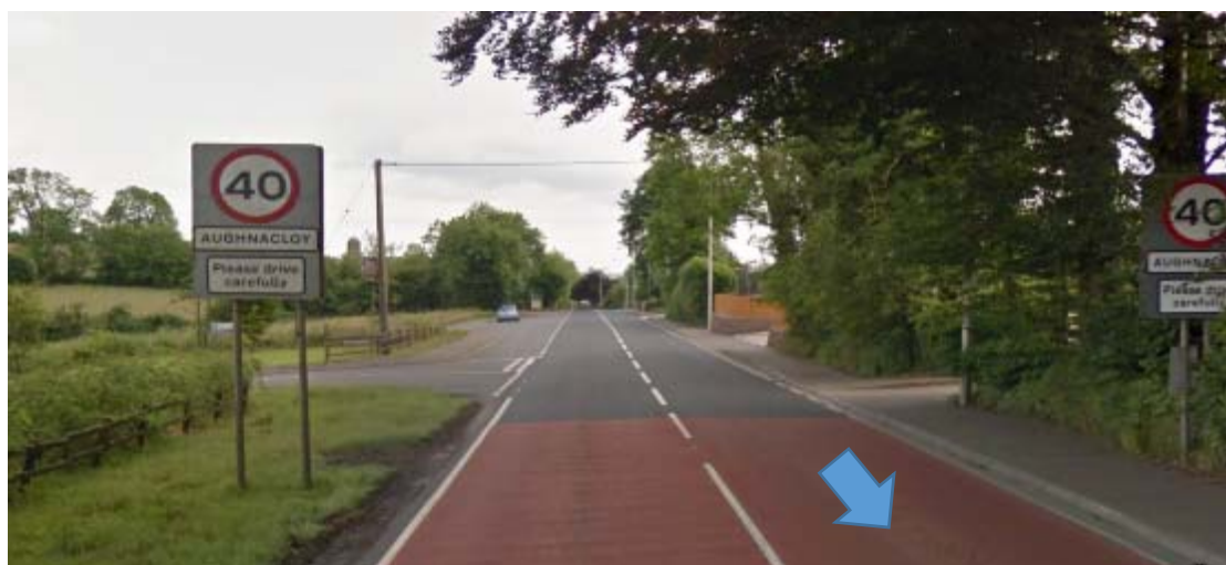
Photograph 5: Potential Shared Use NMU Facility (See Drawing D-029)
