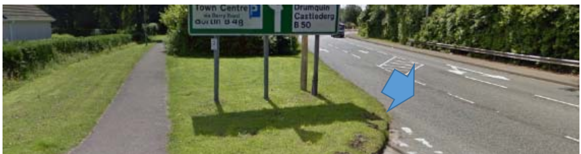
Photograph 26: Northbound view of offline footway between Watson Pk. & Derry Rd. from Derry Rd. (See Drawing D-019)
