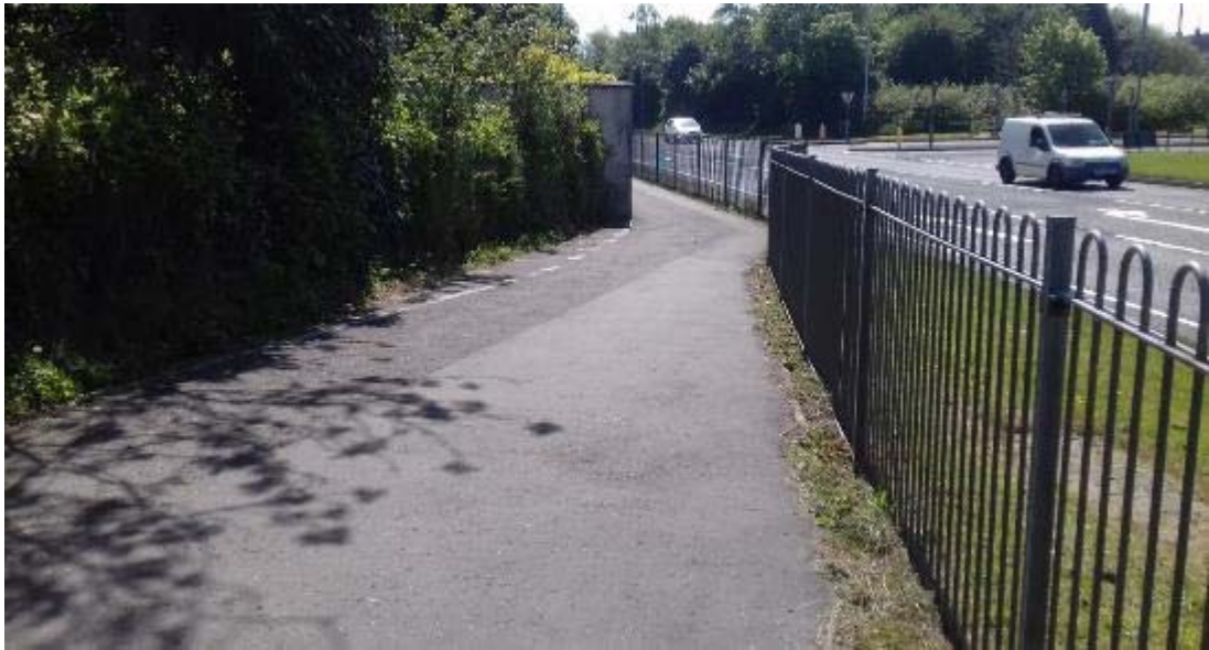
Photograph 35: Offline Footway adjacent to the A5 Great Northern Link (See Drawing D-021)
