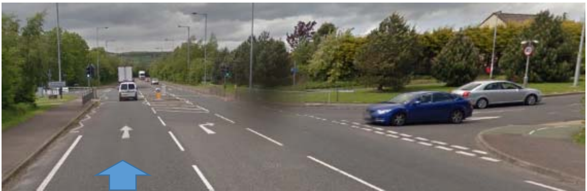
Photograph 10: A5 Great Northern Link south of Orchard Park and Orchard Road exits (See Drawing D-011)
