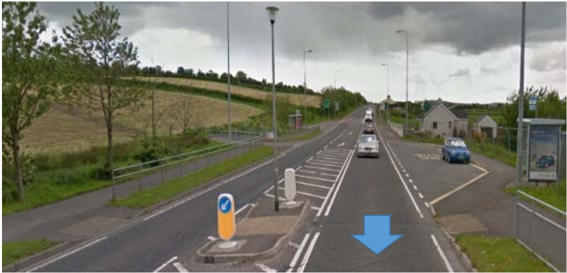
Photograph 4: NMU Crossing with Refuge Island: Approx. 40m south of Victoria Meadows junction with the existing A5 (See Drawing D-003)
