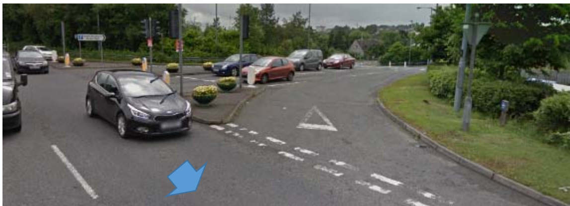
Photograph 12: Tamlaght Rd. exit off the A5 Great Northern Link at the Railway Terrace / Tamlaght Rd. Junction (See Drawing D-022)
