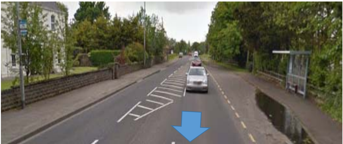
Photograph 14: Southbound on A5 Victoria Road north of New Buildings Primary School (see drawing D-002)
