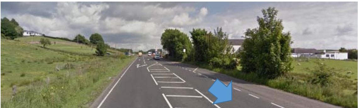
Photograph 5: Southbound on A5 Curr Road, North of Radergan Road (see drawing D-033)
