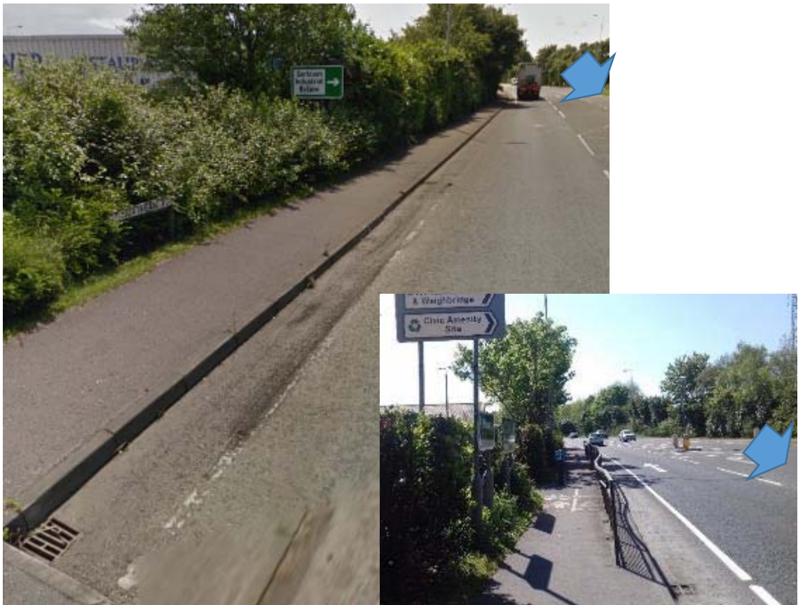
Photograph 5: Left : Southbound view of A5 Great Northern Link exit from Derry Road Roundabout; Right : Southbound view of A5 Great Northern Link opposite the northern entrance to the Gortrush Industrial Estate (See Drawing D-020 for both)
