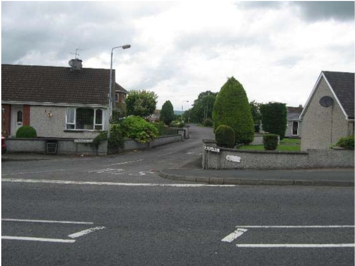
Photograph 8: Uncontrolled Pedestrian Crossing Point (See Drawing D-006)
