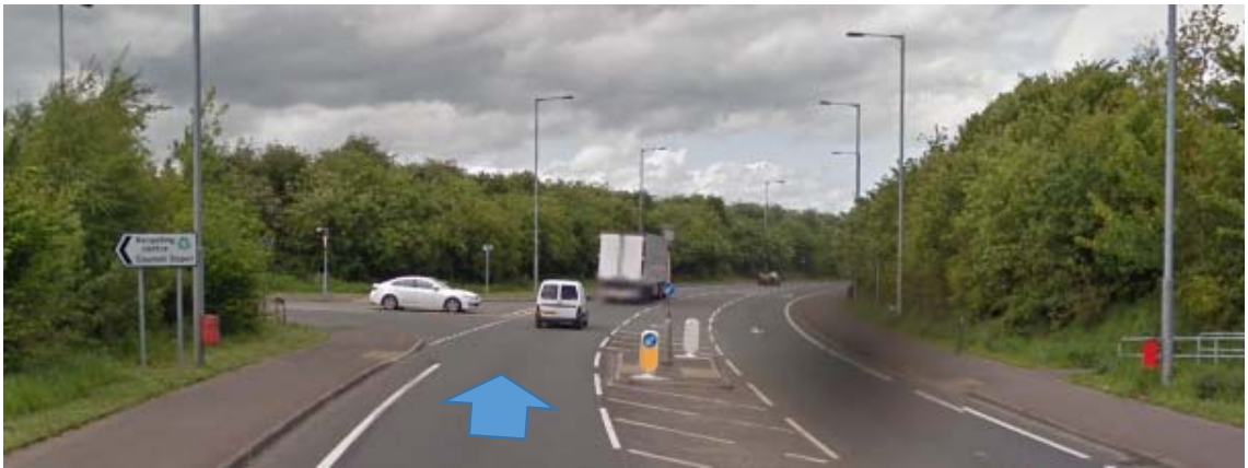
Photograph 9: A5 Great Northern Link south of Strahan Road exit (See Drawing D-011)
