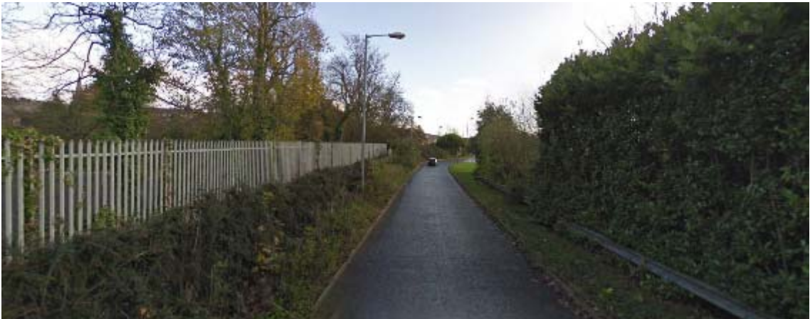
Photograph 37: Southbound on the A5 on-slip from Brook St (See Drawing D-022)
