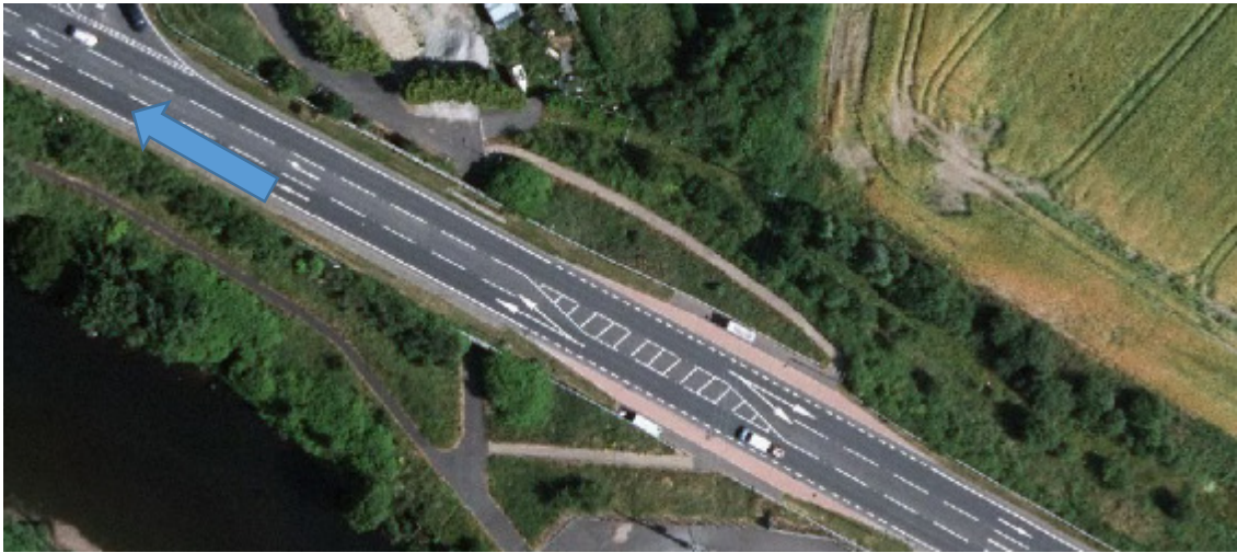
Photograph 5: Widening of existing NMU access to bus stops (See Drawing D-026)
