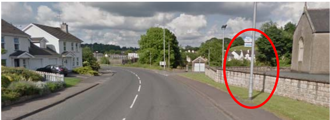
Photograph 8 : Opportunity 2(h) – Addition of Shared Use NMU Facility; Opportunity 5(c) – Addition of Bus Stop Shelter (Red Circle) (See Drawing D-030)
