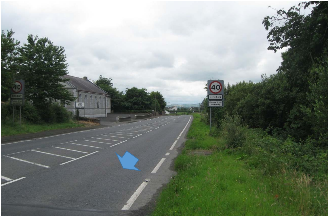
Photograph 2: Southbound entrance to Bready (See Drawing D-004)
