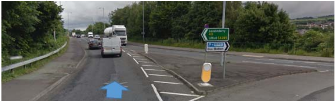
Photograph 3: A5 Northbound exit off the Bradley Way Roundabout (See Drawing D-009)
