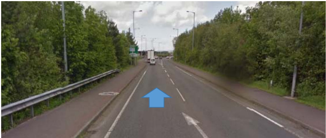
Photograph 7: A5 Great Northern Link south of the junction with Urney Road (See Drawing D-009)
