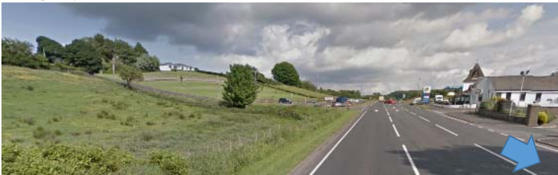
Photograph 6: Southbound on A5 Curr Road north of Radergan Road junction (see drawing D-033)
