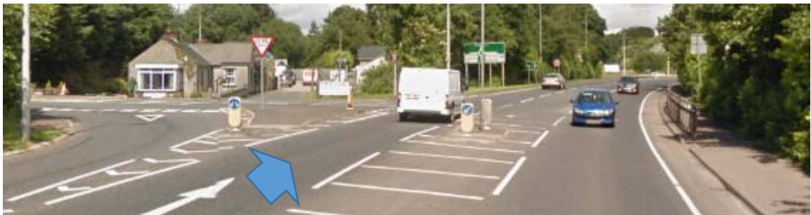
Photograph 7: Northbound view of A5 Great Northern Link south of the entrance to the Gortrush Industrial Estate (See Drawing D-020)
