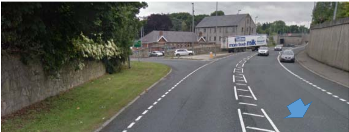
Photograph 43: Southbound on the A5 Great Northern Link immediately north of Dublin Road Exit (See Drawing D-023)
