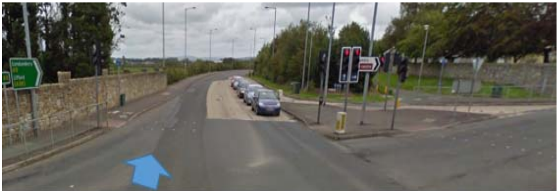
Photograph 6: Northbound on the A5 Great Northern Link at the junction with Urney Road (See Drawing D-009 and D-010)
