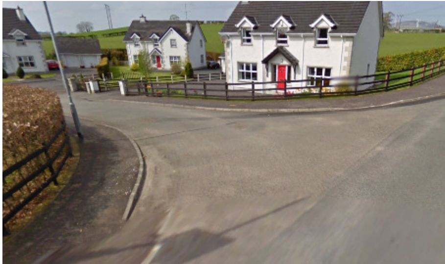
Photograph 3: Uncontrolled Pedestrian Crossing - Castletown Road and Cul-de-Sac (See Drawing D-018)
