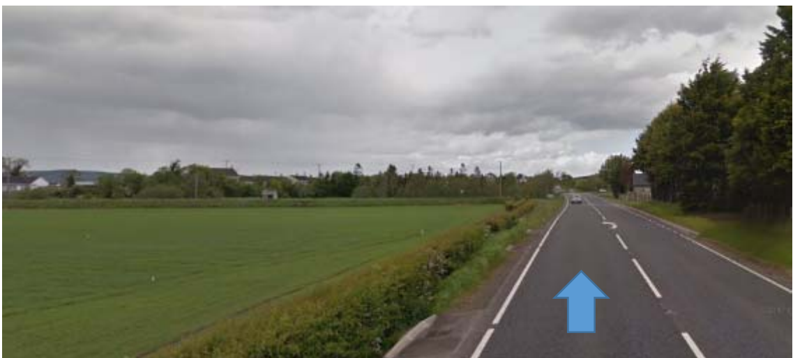
Photograph 6: Northbound entrance to Burndennett (see drawing D-032)
