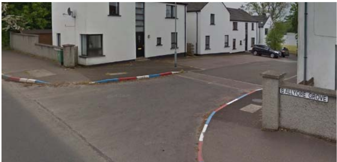
Photograph 10: Ballyore Grove junction with the A5 Victoria Road (see drawing D-002)
