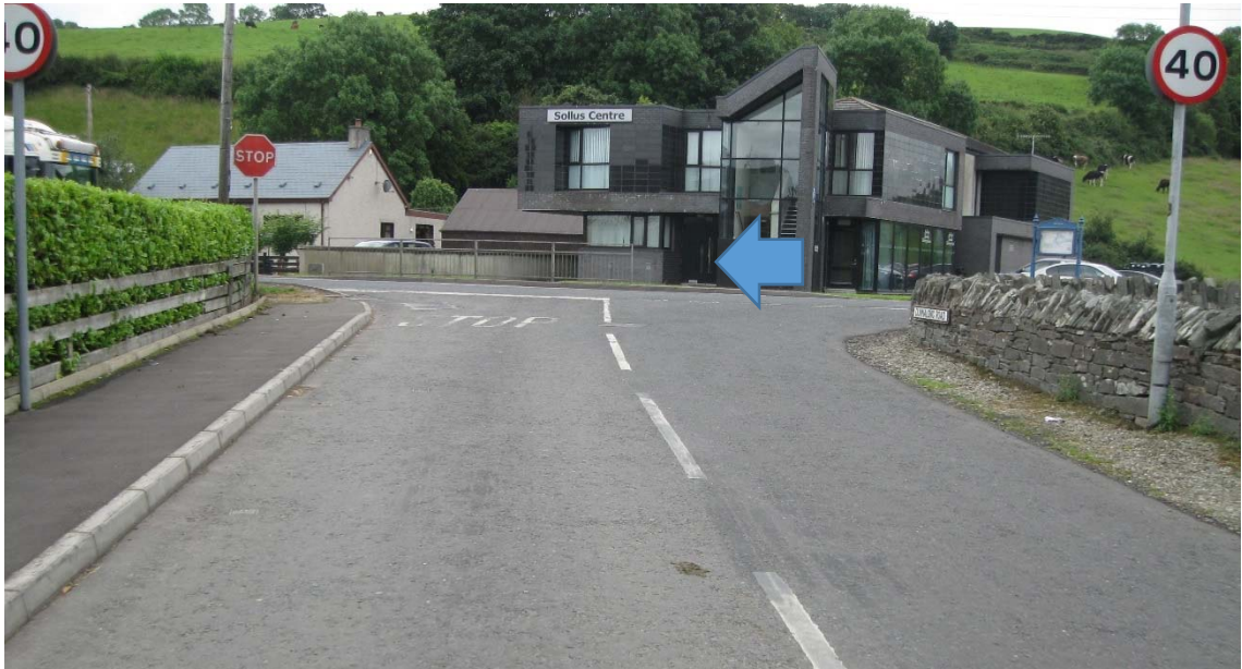
Photograph 6: Dunalong Road approach to A5 Victoria Road (See Drawing D-004)
