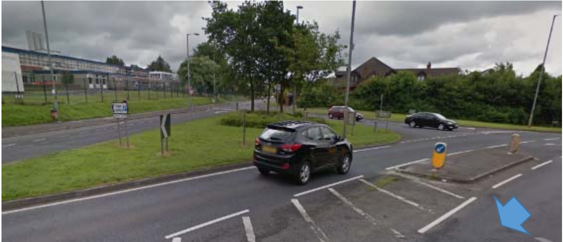
Photograph 23: A5 Derry Road north junction with Derry Road (See Drawing D-007)
