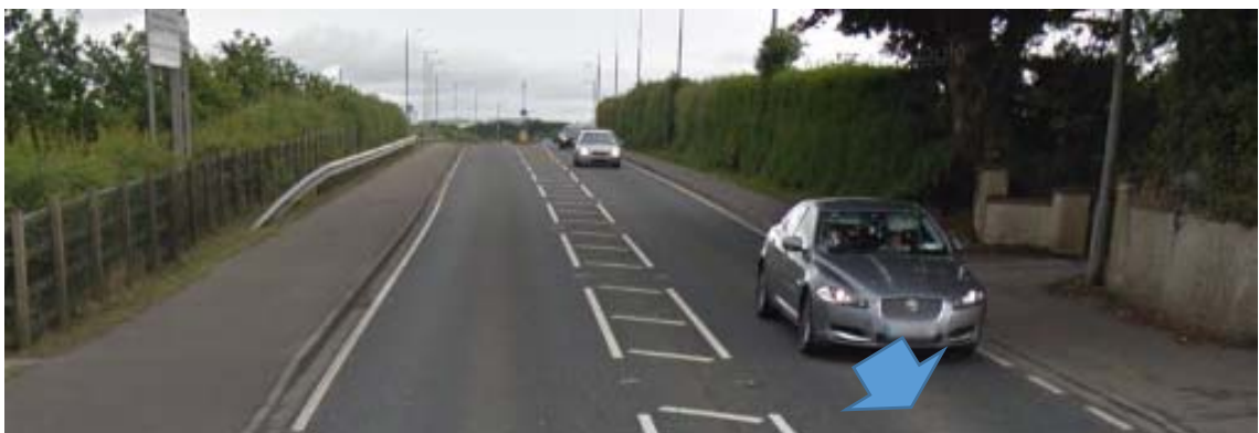
Photograph 20: A5 Melmound Road south of the entrance to the Strabane Business Park (See Drawing D-011)
