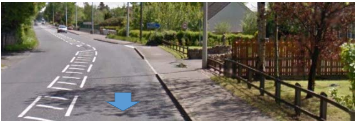
Photograph 19: Southbound footway extension to the entrance to Omagh Rugby Club (See Drawing D-019)
