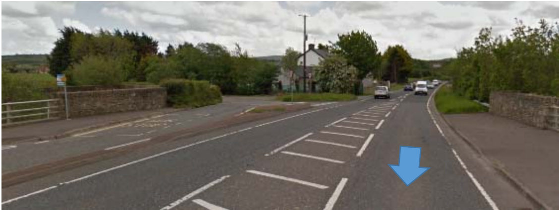
Photograph 2: Uncontrolled NMU Crossing (see drawing D-032): Burndennett Overbridge Structure
