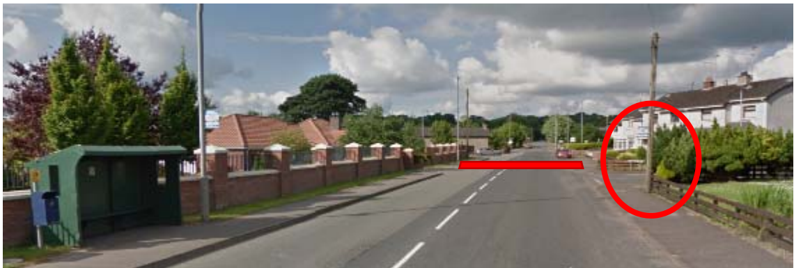
Photograph 14: Opportunity 5(d) – Addition of Bus Stop Shelter (Red Circle) Opportunity 3(p) – Uncontrolled Pedestrian Crossing (Red Rectangle) (See Drawing D-030)
