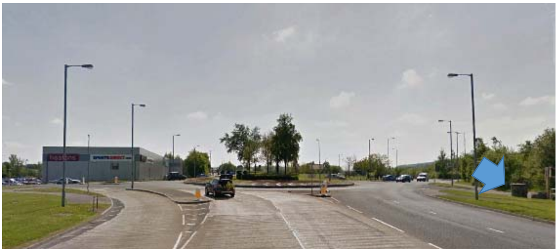
Photograph 14: Existing Pedestrian Refuge Island: A5 Barnhill Road at Roundabout Junction, Lifford Road and Railway St. (See Drawing D-008)
