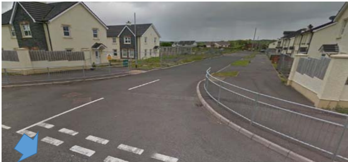
Photograph 3: Existing Uncontrolled Pedestrian Crossing: Victoria Meadows junction with the A5 (See Drawing D-003)
