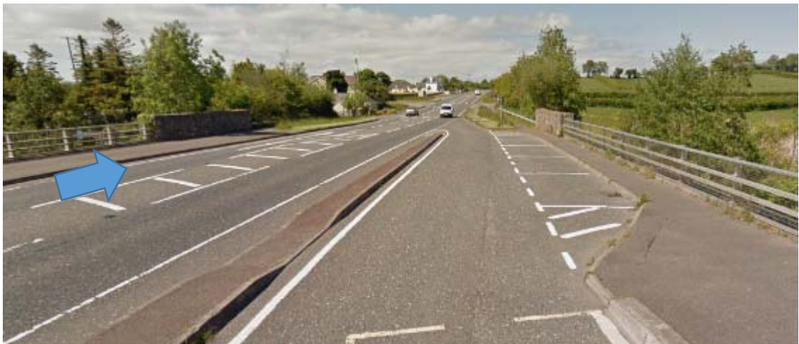
Photograph 1: Existing parking facilities on Burdennett Overbridge Structure (see drawings D-032)
