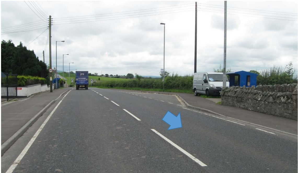
Photograph 7: A5 Victoria Road south of the Dunnalong Road exit (See Drawing D-004)
