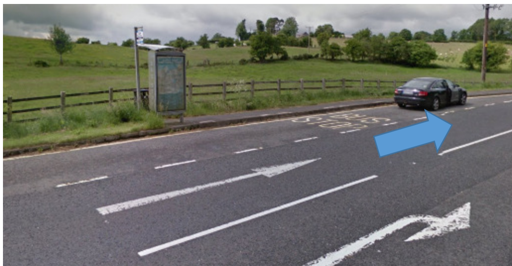
Photograph 4: Larger Bus Stop shelter (northbound) outside Folk Museum (See Drawing D-017)
