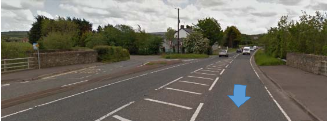
Photograph 9: Southbound on A5 Victoria Road, existing NMU crossing facility upgrade (see drawing D-032)
