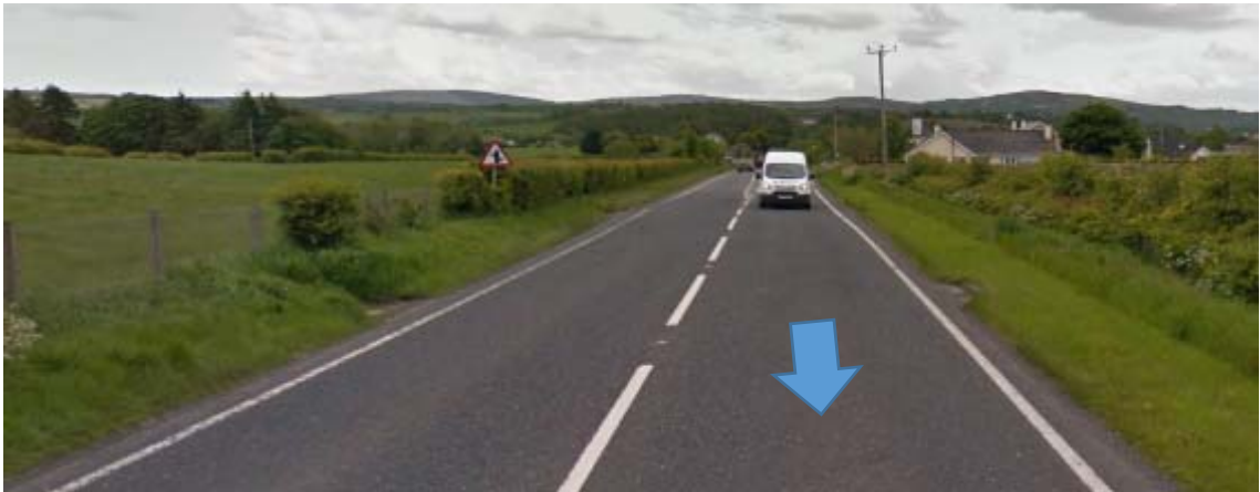
Photograph 12: Southbound on A5 Victoria Road south of Ash Avenue junction (see drawing D-031 and D-032)
