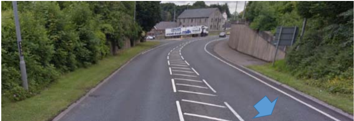
Photograph 42: Southbound on the A5 Great Northern Link north of Dublin Rd. Exit (See Drawing D-023)
