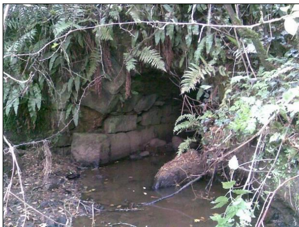
Photograph 3.3.2-3 - Augher Road Bridge (North) on the River Letfern - Upstream view (GR 250601, 364275)
