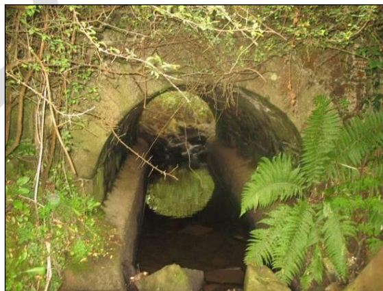
Photograph 3.2.8-5 – Fireagh Lough Drain at Brookmount Road
