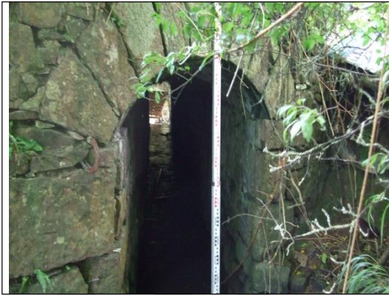
Photograph 3.3.13-3 - Main Channel Stone Masonry Spring Arch at Carnteel Road
