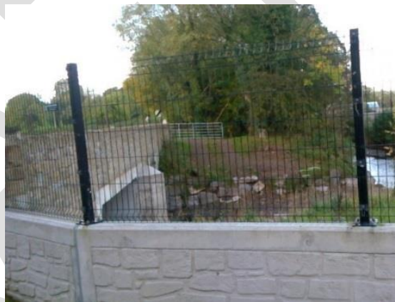
Photograph 3.3.9-4 - Tullybryan Road Bridge upstream flood defences
