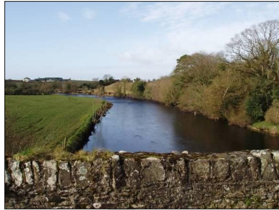
Photograph 3.2.2-2 – Derg River Upstream of Old Bridge Road
