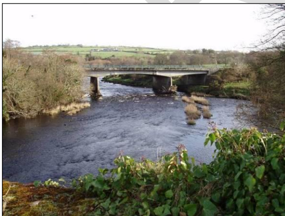
Photograph 3.2.2-3 – Strabane Road Bridge at Millbrook
