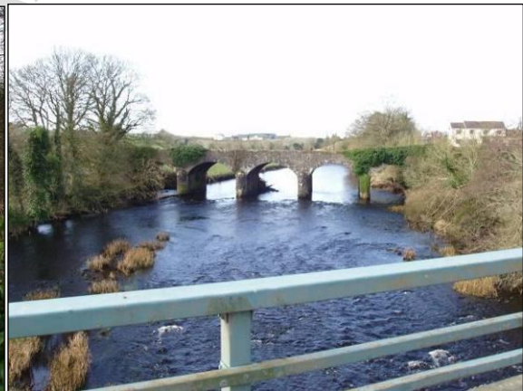
Photograph 3.2.2-4 – Old Bridge at Mill Brook
