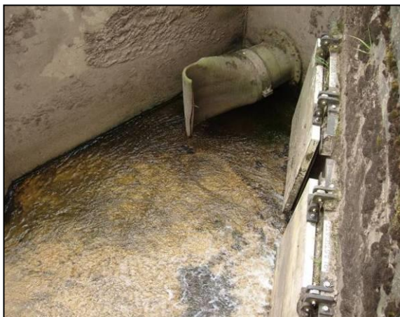
Photograph 3.2.7-5 – Outfall of Hunters Crescent Stream into River Strule
