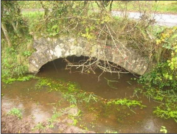
Photograph 3.3.6-1 - Culvert under Newtownsaville Road
