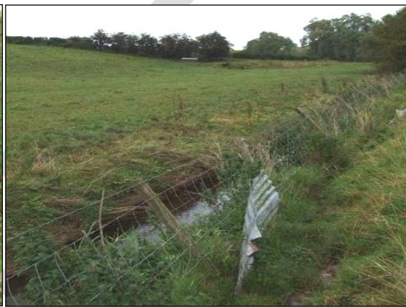
Photograph 3.3.1-2 - Ranelly Drain Typical Channel
