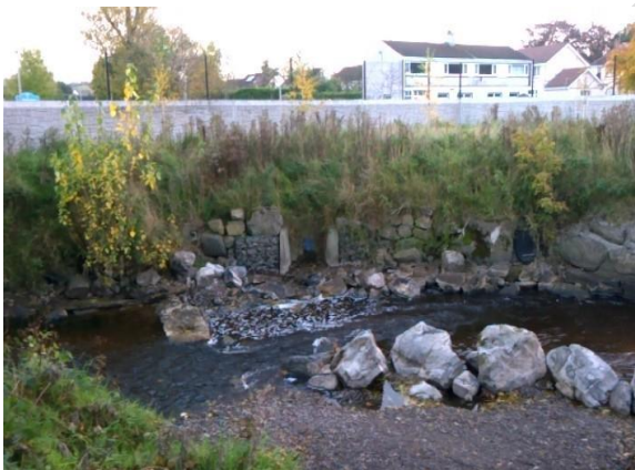
Photograph 3.3.9-3 - Tullybryan Road Bridge adjacent flood defences
