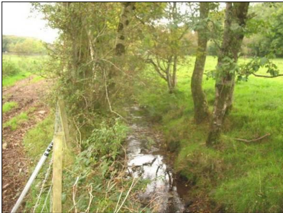
Photograph 3.2.8-3 – Fireagh Lough Drain; North of Clanabogan Road
