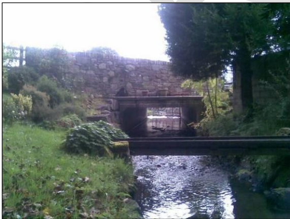
Photograph 3.3.2-1 - Augher Road Bridge (North) on the River Letfern - Upstream View (GR 250601, 364275)
