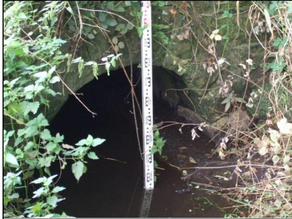
Photograph 3.3.13-7 South Tributary Stone Masonry Arch at Field Access Track
