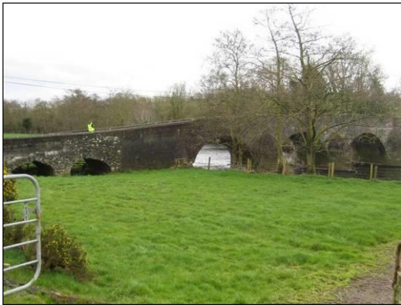
Photograph 3.2.9-3 – Drumragh Bridge and Flood Relief Arches
