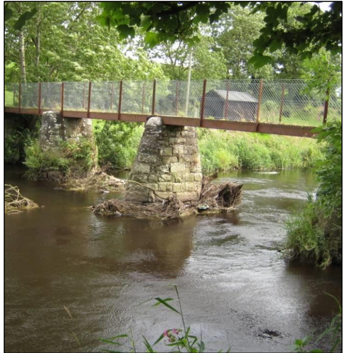
Photograph 5.3.9-2 – Drumshanly steel footbridge
