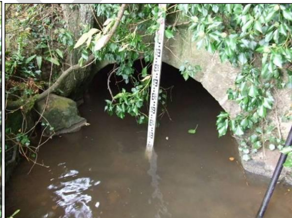
Photograph 3.3.13-4 - Main Channel Stone Masonry Arch at Rehaghy Road
