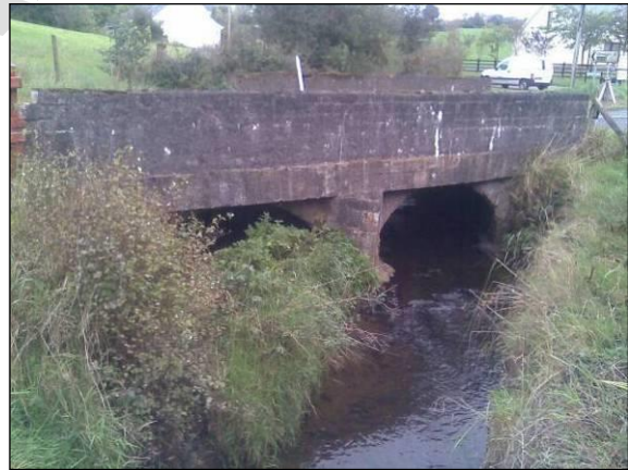
Photograph 3.3.2-2 - Moylagh Road Bridge on the River Letfern - Upstream View (GR 250595, 364205)
