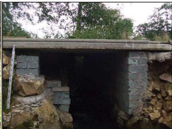
Photograph 3.3.13-6 - North Tributary Brick Masonry Bridge at Field Access Track
