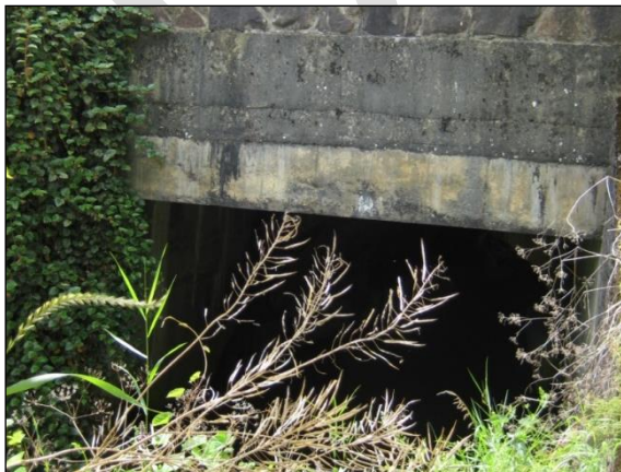
Photograph 3.3.13-5 - Main Channel Concrete Culvert at Monaghan Road
