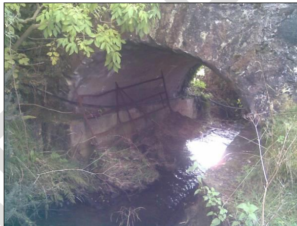
Photograph 3.2.6-3 – Lisnagirr Road Bridge
