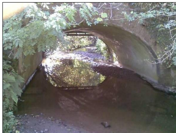
Photograph 3.3.8-4 - Arch of Ballynasaggart Bridge
