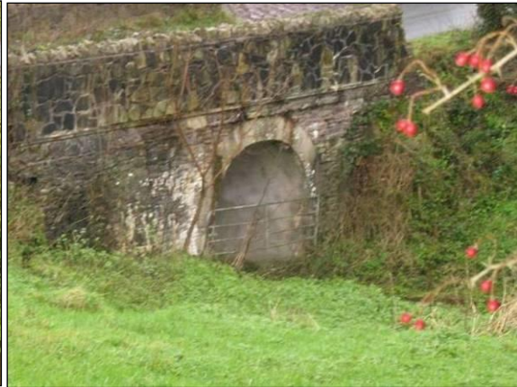
Photograph 3.3.6-2 - Bridge under Springhill Road
