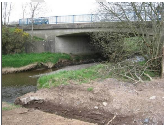
Photograph 3.3.9-5 - Annaghilla Road Bridge
