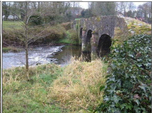
Photograph 3.2.9-4 – Lissan Bridge and Downstream Weir
