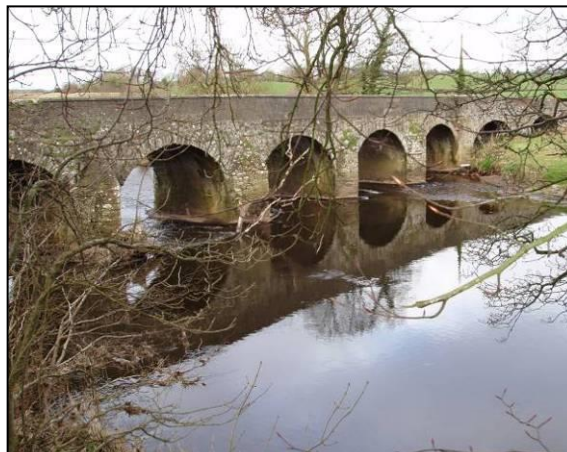
Photograph 3.2.7-6 – Downstream model boundary at Tattracnaghty stone bridge
