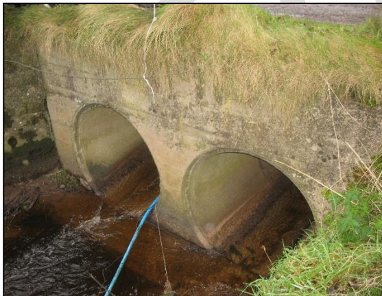
Photograph 3.3.1-3 – Tullyrush Road Culverts on the Ranelly Drain - (GR 248818 366252)
