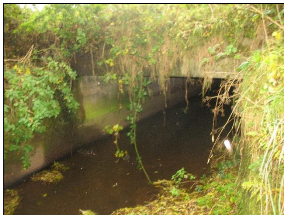
Photograph 3.3.1-5 – Doogary Road Culverts on the Ranelly Drain - (GR 248425 367872)
