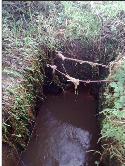
Photograph 3.3.3-3 – 200mm dia pipe culvert located in the Northern tributary
