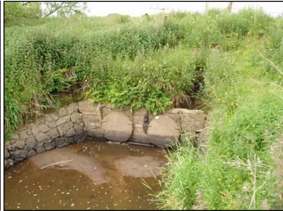
Photograph 3.2.7-2 – Outfall of Tully Drain at confluence with River Strule
