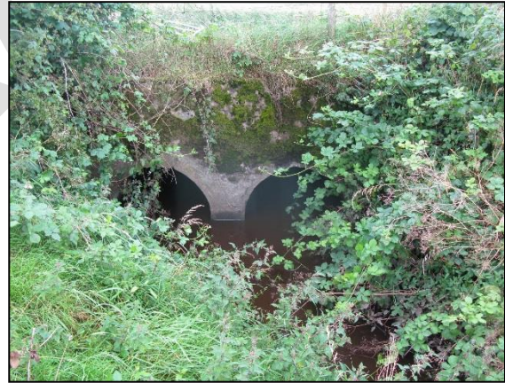
Photograph 3.3.1-4 – Access Track Culverts on the Ranelly Drain - (GR 248331 367303)
