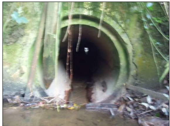
Photograph 3.3.9-6 - 900 mm Culvert Underneath Annaghilla Road
