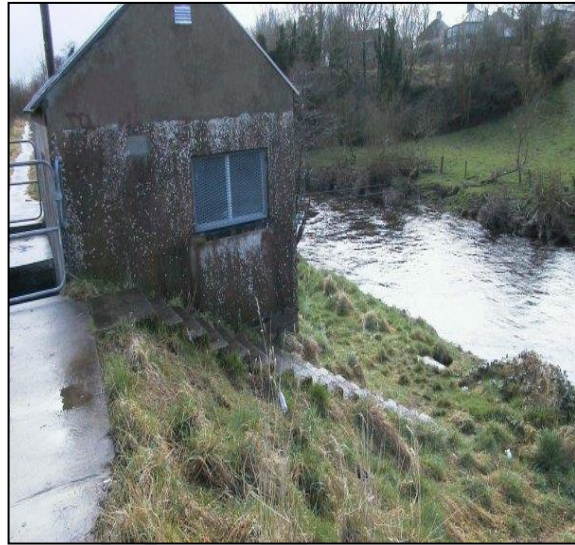
Photograph 5.3.9-4 – Campsie Bridge gauging station
