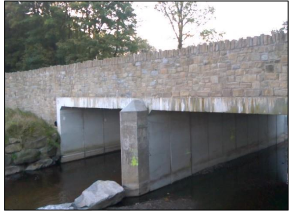
Photograph 3.3.9-2 - Tullybryan Road Bridge
