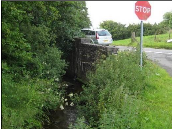
Photograph 3.3.7-3 - Tycanny Road Bridge
