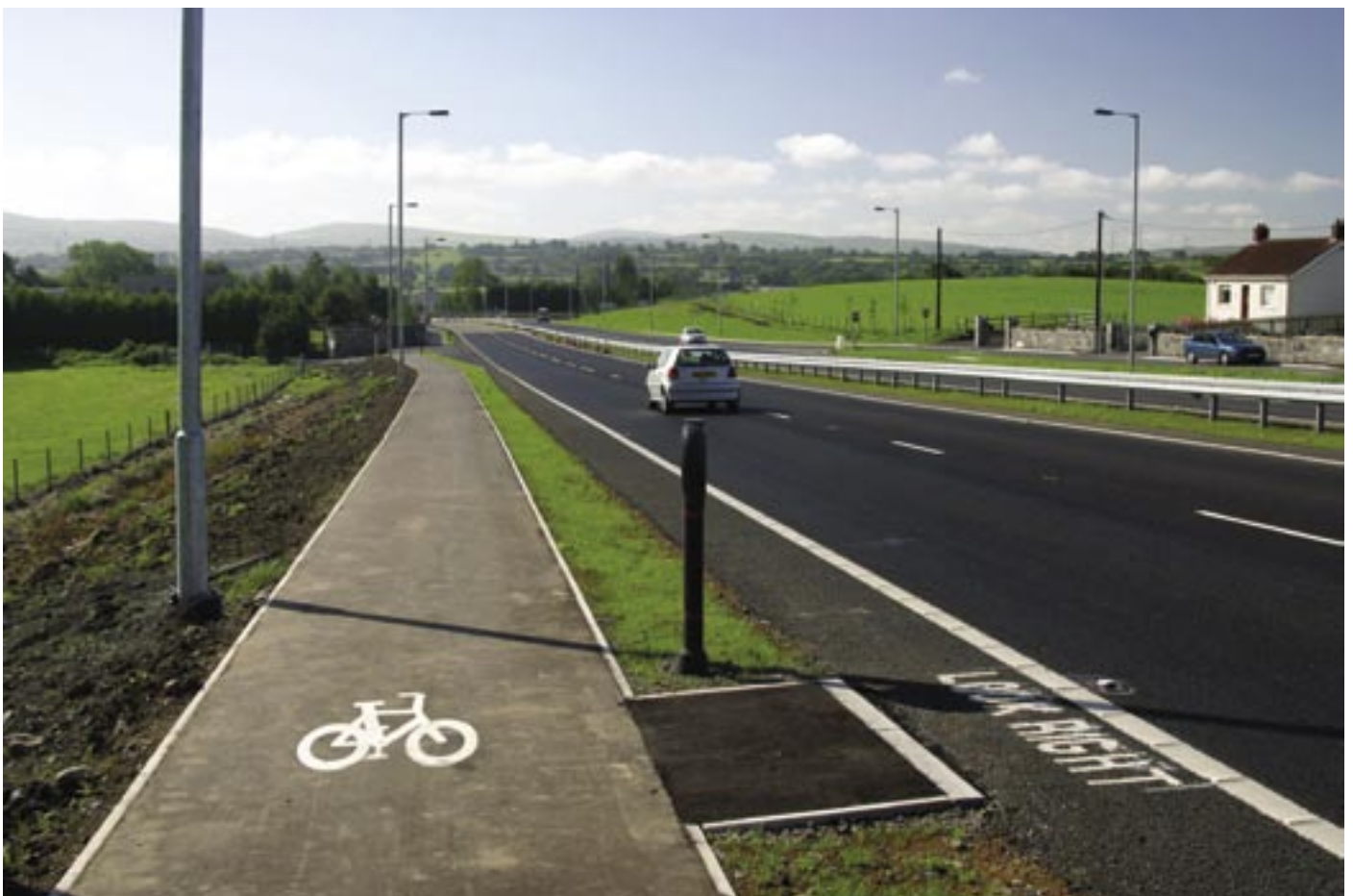
Cycling facilities along the A8 Belfast - Larne Road Dualling
