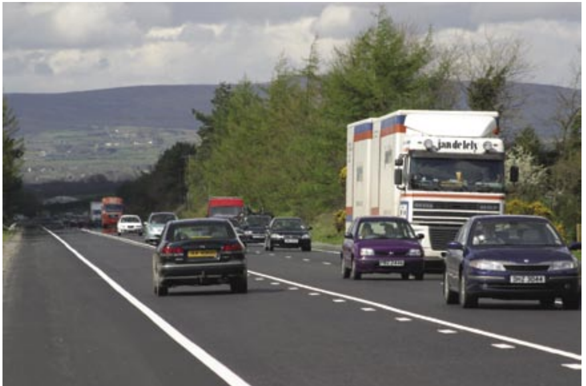
Widened single carriageway, Curran
