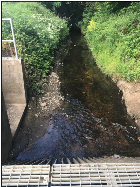
Picture 3.3 Channel immediately upstream of culvert inlet
