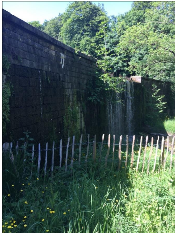
Picture 3.1 Dungannon Park Lake Dam Wall
