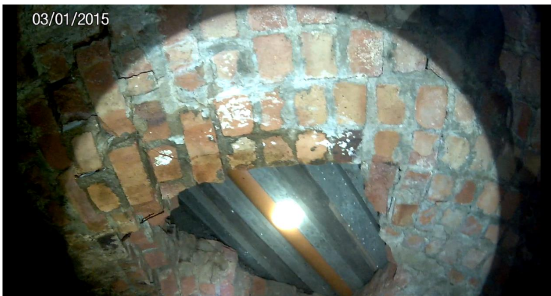
Picture 9.2 Missing bricks in roof of culvert near manhole U4304/06
