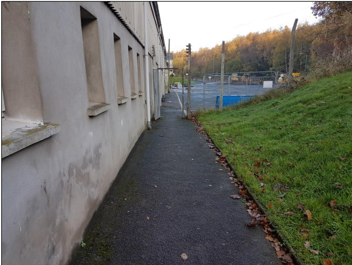
Picture 6.3 Windows along eastern side of Transport NI Garage
