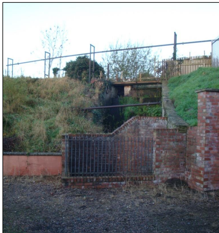
Picture 3.5 Outlet Sluice, Overflow and Cascade at Linen Green
