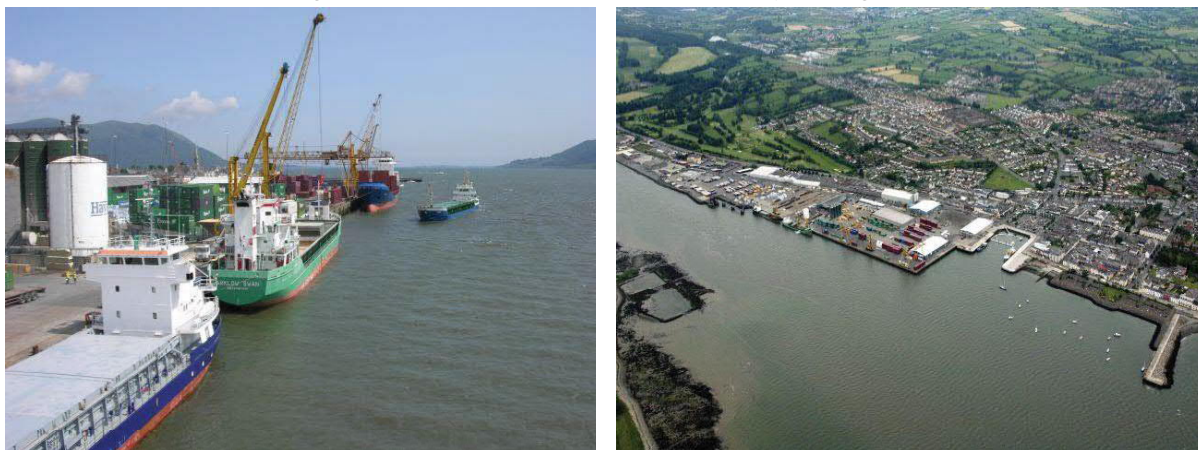
Figure 2.2.1 – Cargo handling and Aerial Photography of Warrenpoint Port
