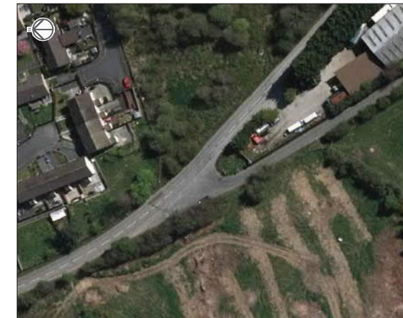
B79 DRUMALANE ROAD / HILLHEAD ROAD
