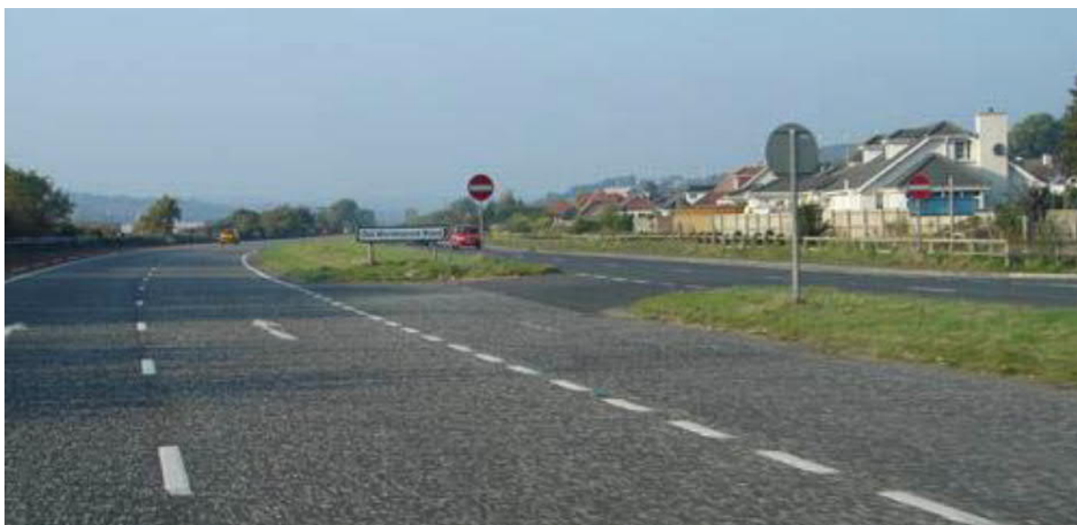
Figure 2.3.4 – A2 Warrenpoint Road (Image showing gap/cross over type junction)
