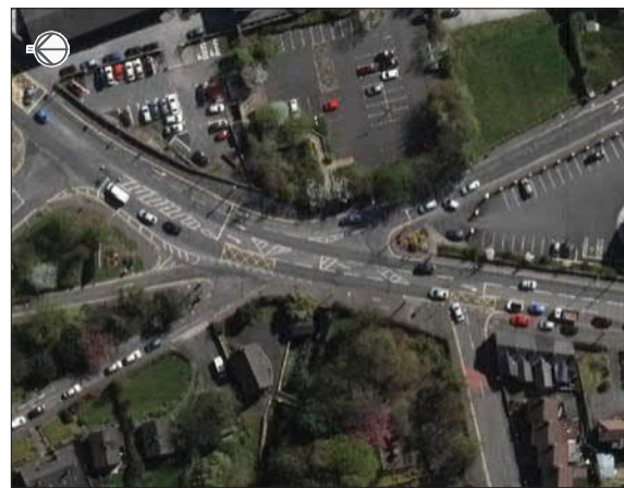
DUBLIN ROAD / DRUMALANE ROAD / DOMINIC STREET
