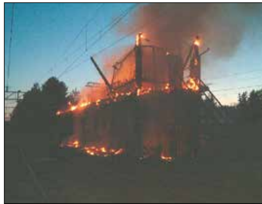
Figure 5: Signal box fire (deliberate fire setting)
