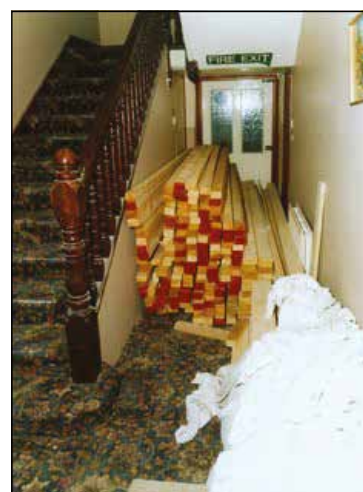
Figure 9: A blocked corridor with incorrect signage
