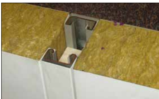
Figure 17: Insulated core panels - internal panel
