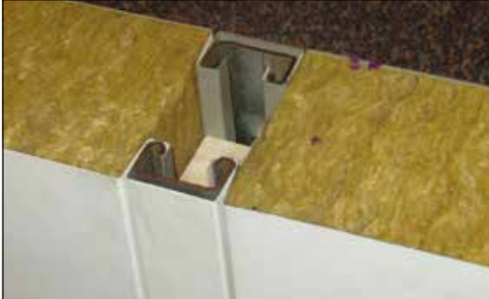
Figure 17: Insulated core panels - internal panel
