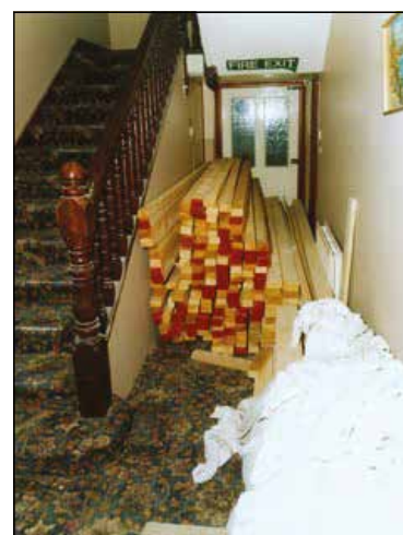
Figure 9: A blocked corridor with incorrect signage
