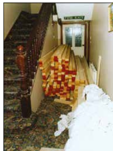
Figure 9: A blocked corridor with incorrect signage
