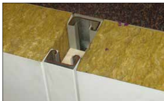
Figure 17: Insulated core panels - internal
