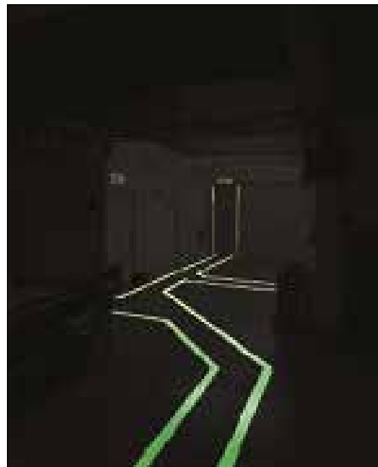
Figure 58: A "way guidance" system
