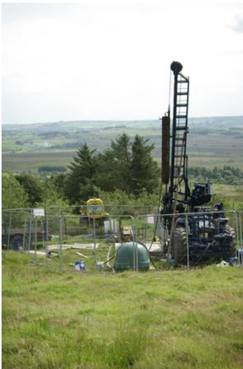
Exploration drill rig
