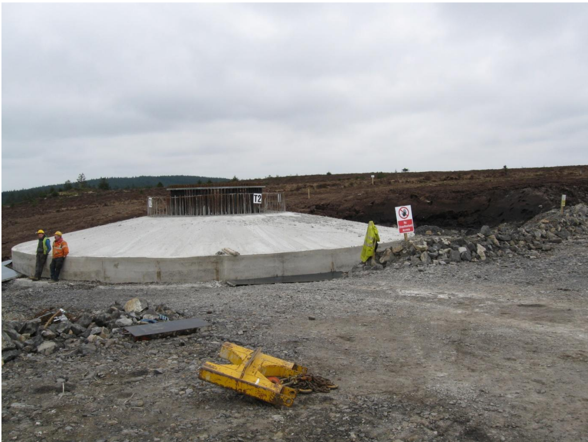
Figure 1: Construction of the foundation of a single wind turbine.
