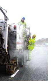
The process of removal using a road planer changes the physical nature of the material from a continuous homogeneous body to a granular material by milling. There is no chemical change to the material when using this process.
