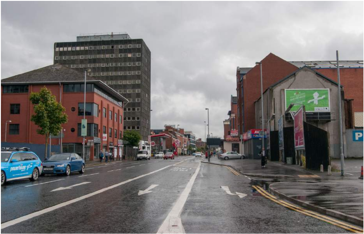
The view along Great Victoria St., back towards Shaftesbury Sq. from Hope St. This image demonstrates how unappealing this street has become, created by ill-mannered buildings and public realm, gap sites and vacancy.
