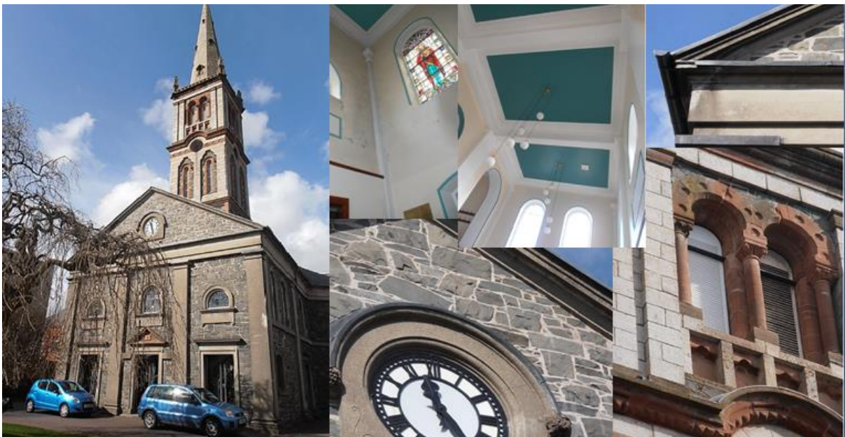
1 st Presbyterian Church Bangor – stone repairs
