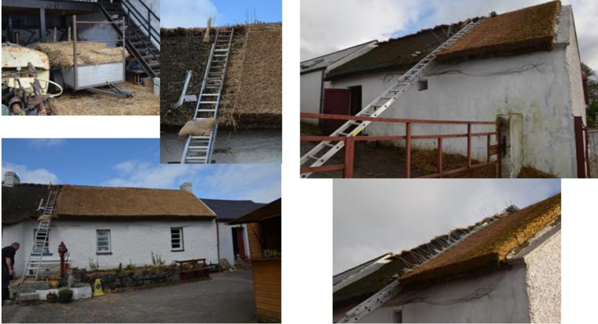
Thatching at Dan Winter's cottage
