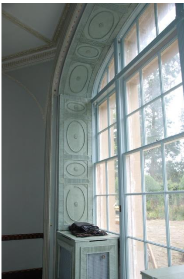
Repairs to window and linings Mount Stewart
