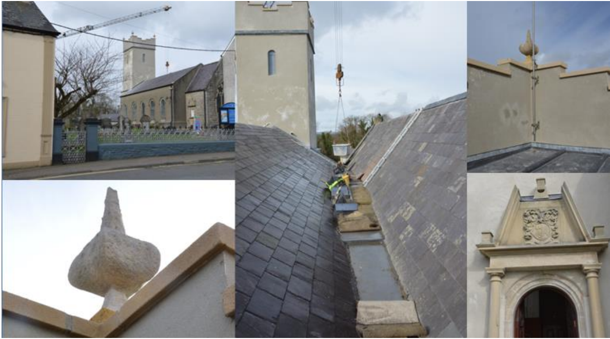
Derg Parish Church Castledearg – roof repairs
