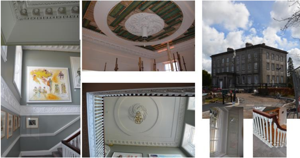
Bishop's Palace Armagh – repairs to interior plasterwork
