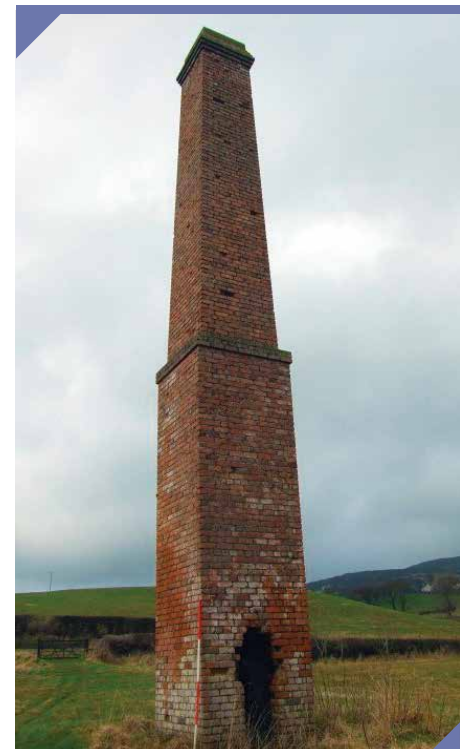
Deehommed, Co. Down flax mill chimney, Photo: NIEA
