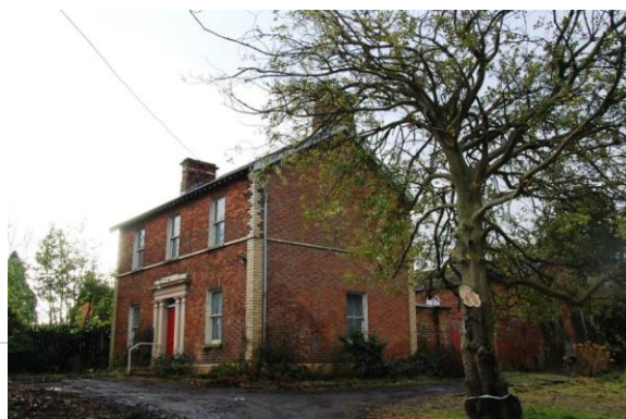
Left: Navigation House, 134 Hillsborough Road, Lisburn © DfC
