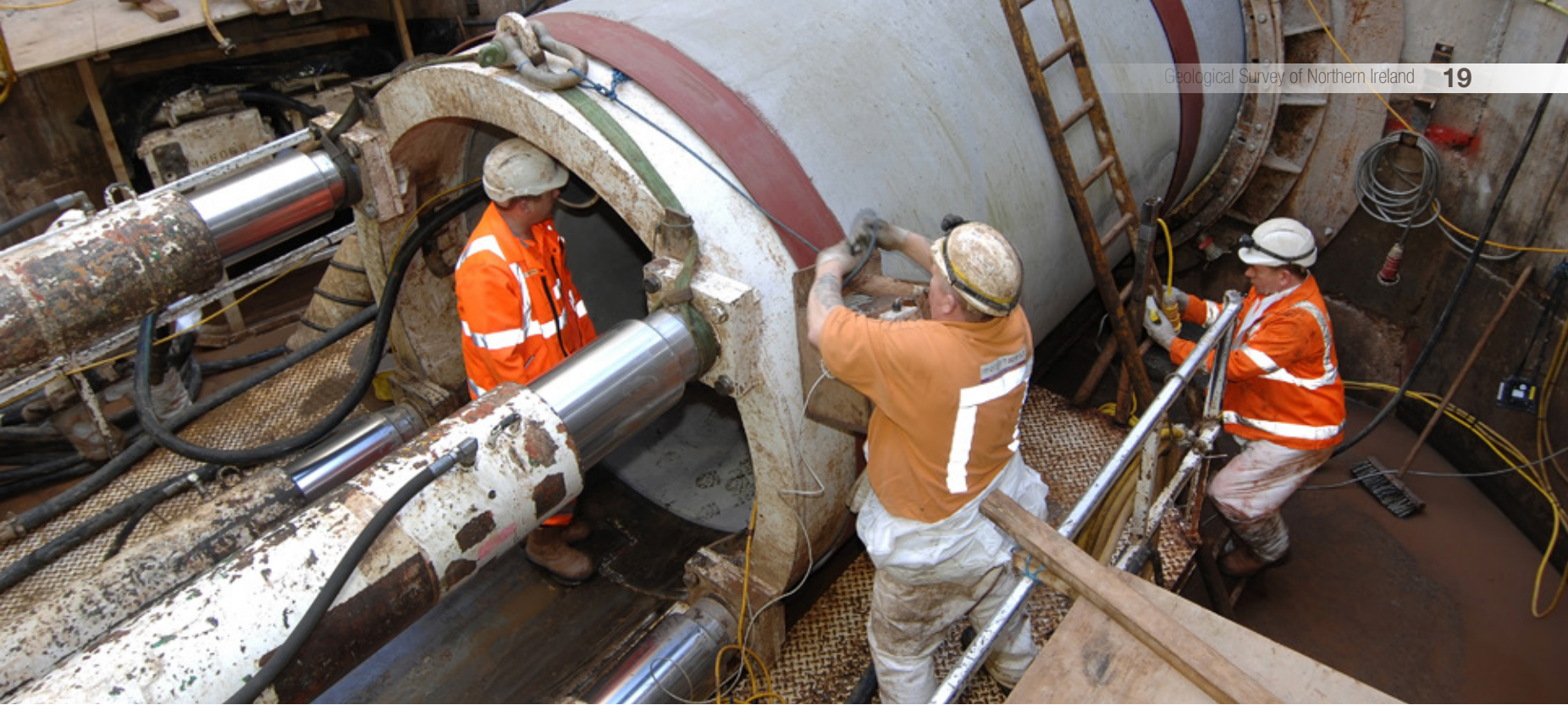
Work on the Belfast sewers project. Courtesy of Akins.
