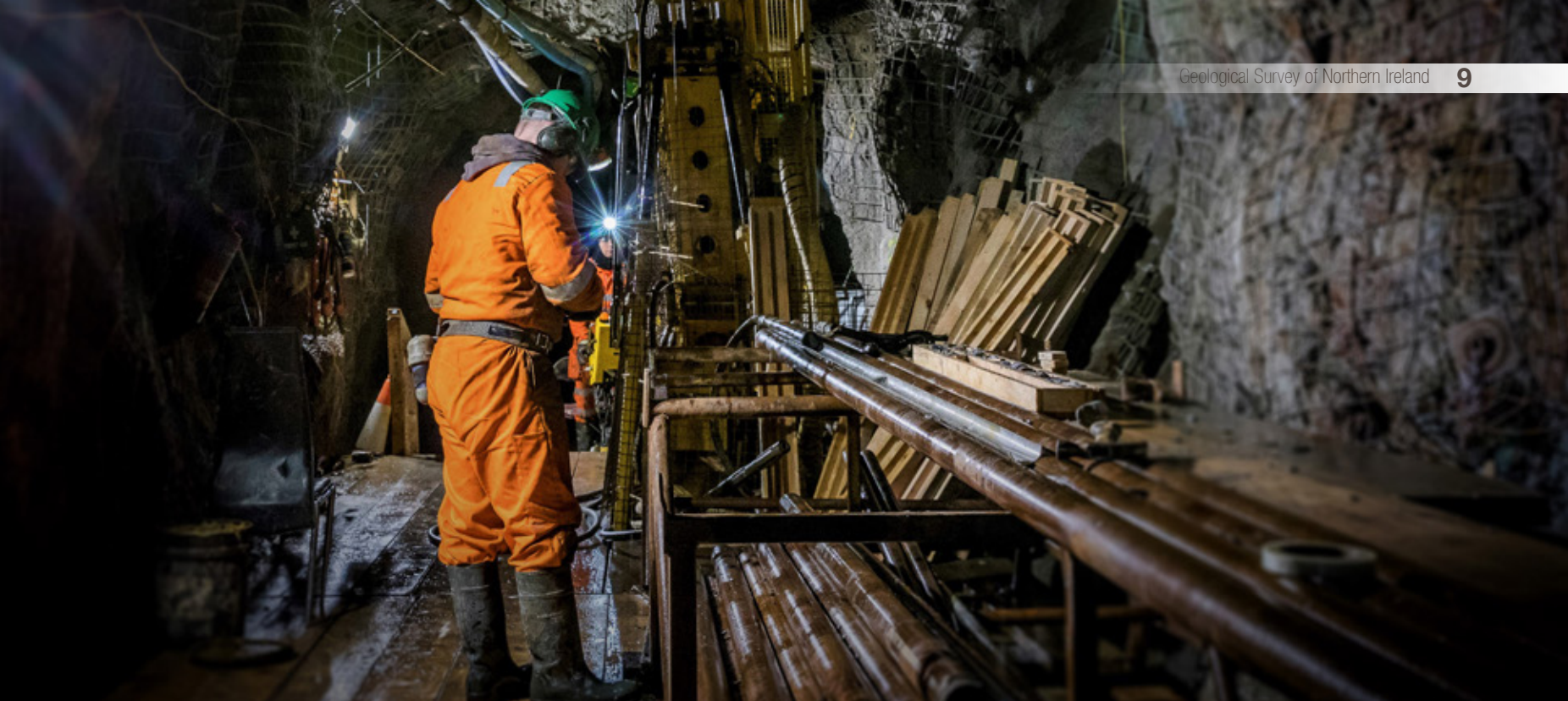
Underground at the Curraghinalt gold deposit. Courtesy Dalradian Gold.
